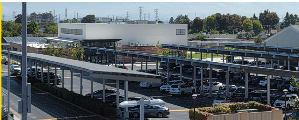
Solar Panels at San Mateo High School
