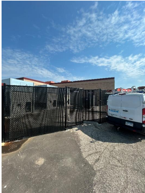
Chiller Screen Replacement
