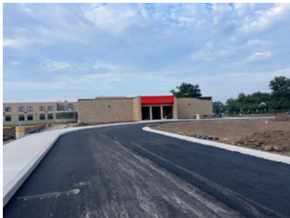
A paved entry loop at the new UPK addition.
