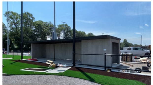
Pre-fabricated dugouts were installed.
