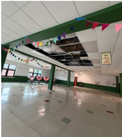
Air conditioning was installed at Smallwood cafeteria.
