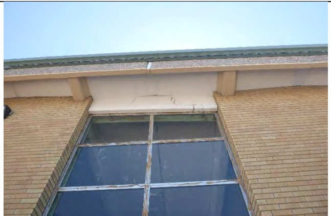
Photo 2 – Concrete beam cracking over NW gym window (7/20/2022).
