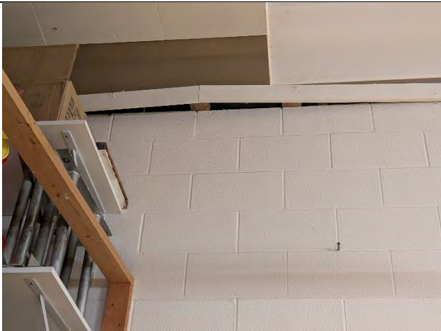
Photo 3 – Concrete beam cracking over NW gym window (1/30/2026).
