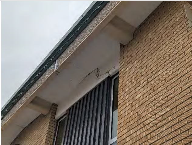
Photo 1 – Concrete beam cracking over NW gym window (1/30/2026).
