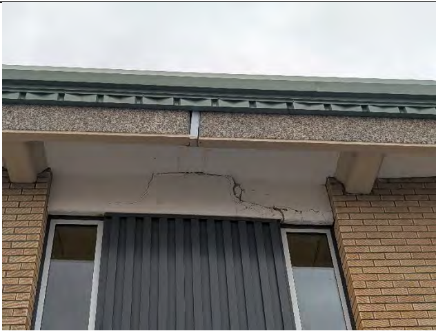
Photo 1 – Concrete beam cracking over NW gym window (1/30/2026).
