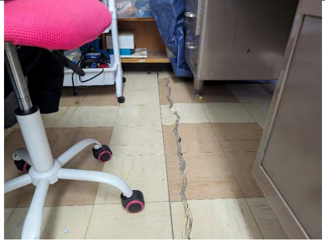
Photo 8 – Floor cracking/movement between concrete T-beams in classroom (1/30/2026).
