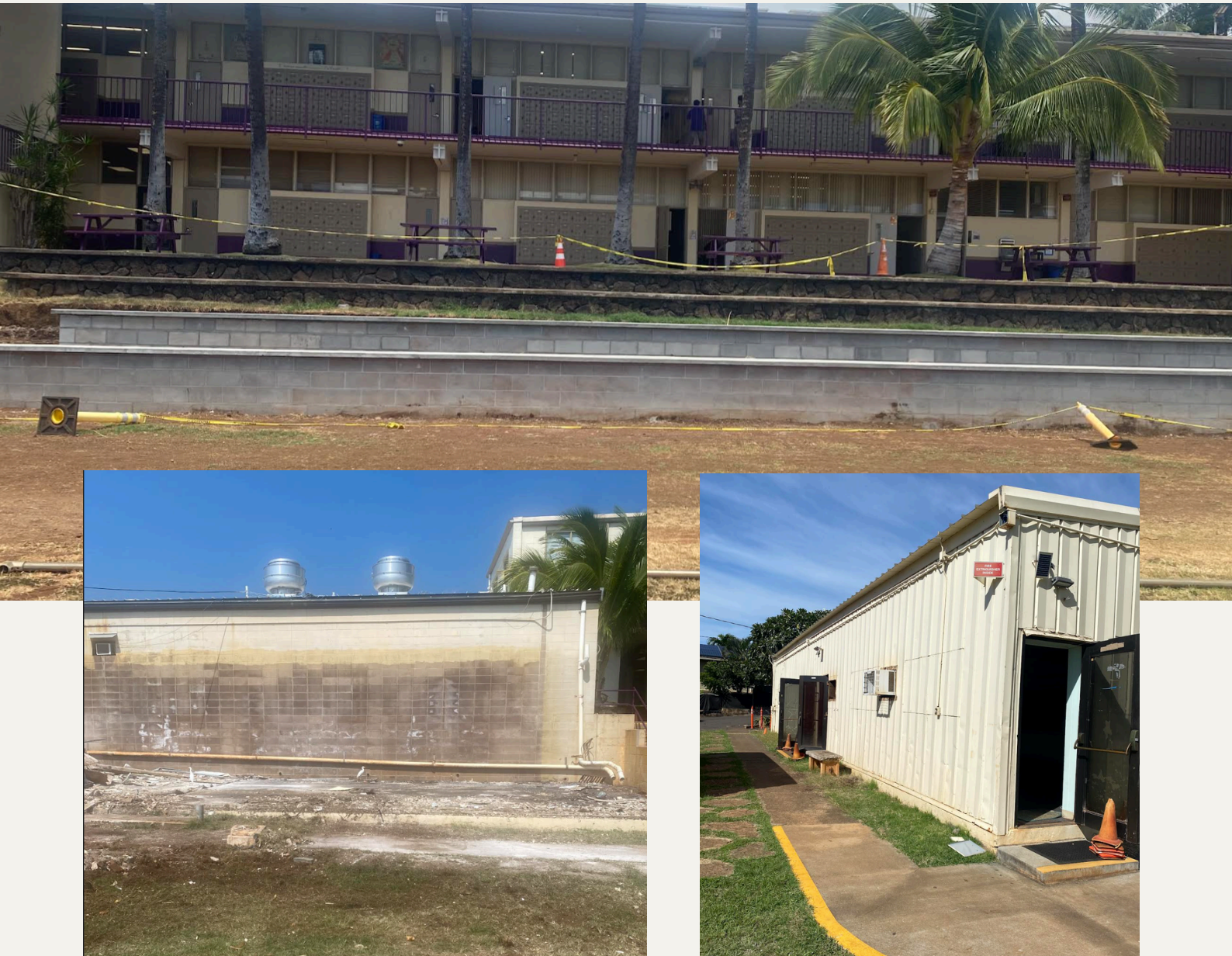
Current progress of DeVeuster Multi-purpose Field.
