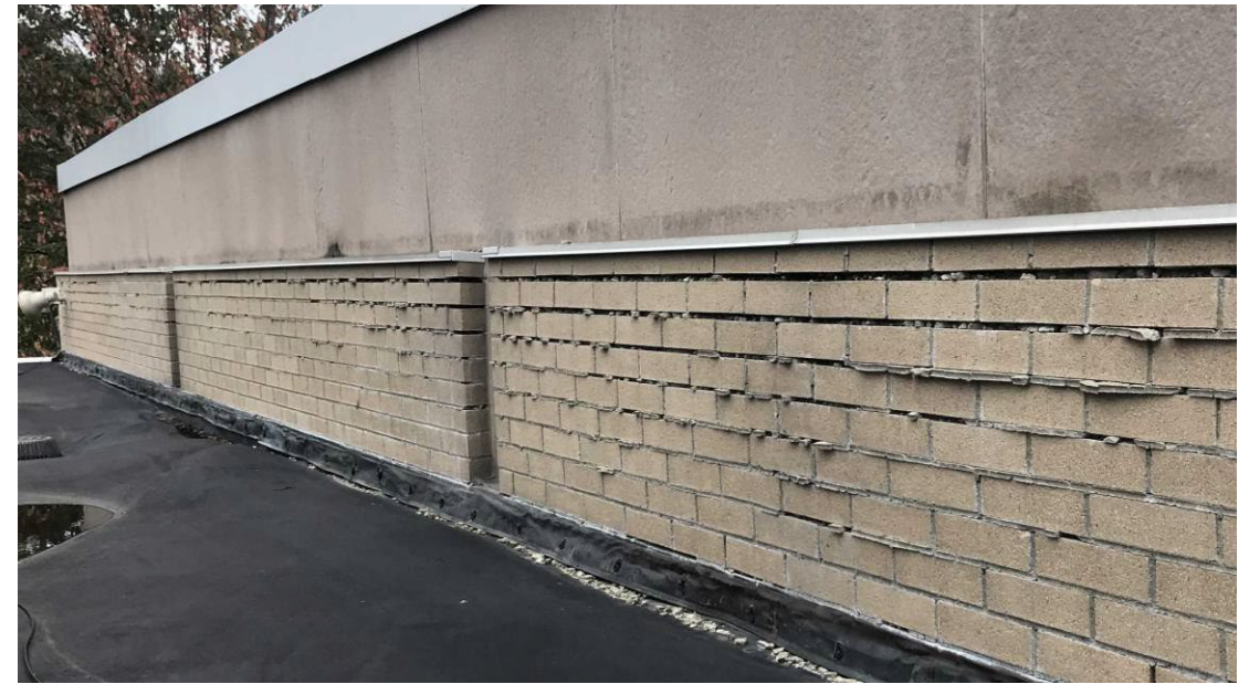
Repairs to Exterior Walls (Wall above Pool Fan Room shown here)
