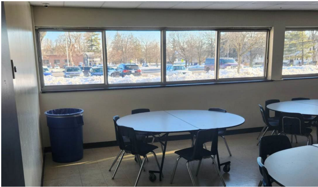
Replace Cafeteria Windows (Cafeteria C shown here)
