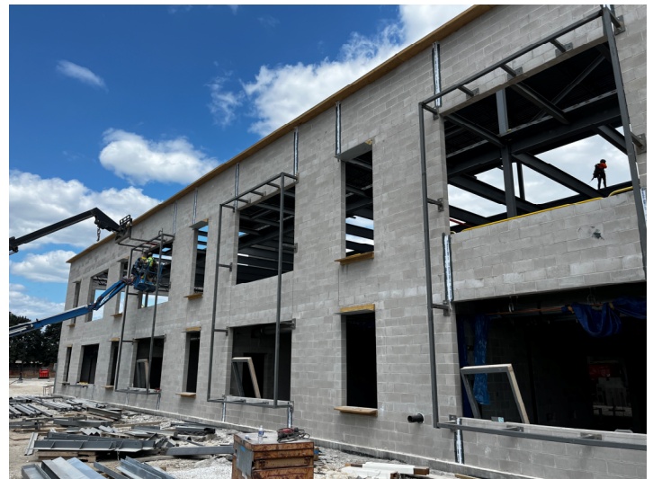
Cold Steel Framing – Area C1 – South Elevation
