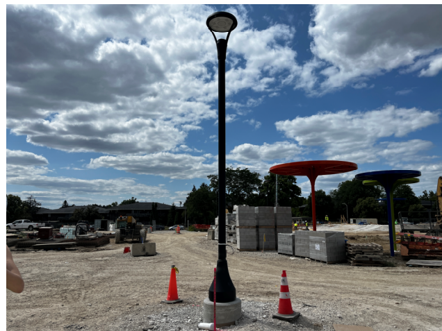
Light Poles Installed – Site
