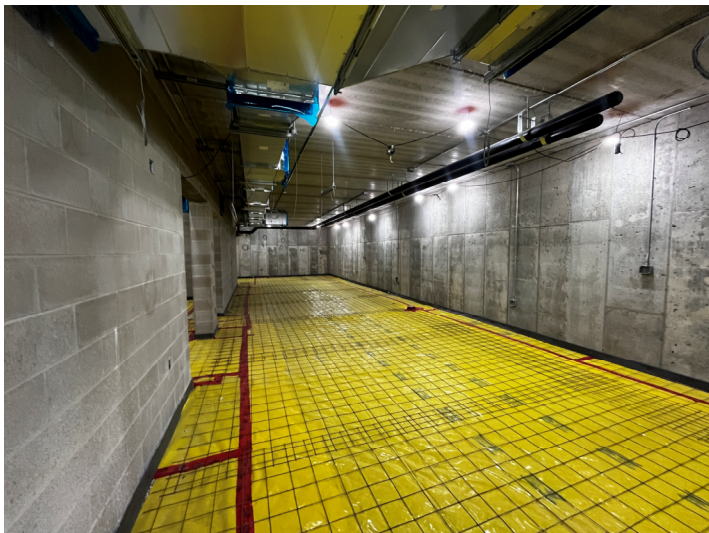
Prepping For Concrete Pour – Area B1 Ground Level
