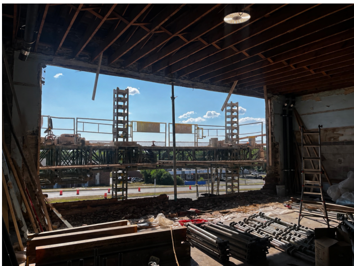
Rework Of An Opening – Area A1 3 rd Floor East Elevation
