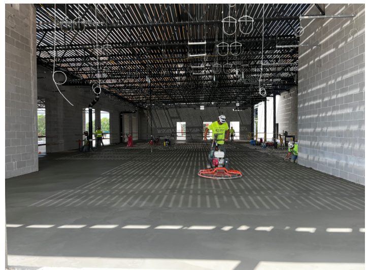
Concrete Poured – Area B1 – 1 st Floor
