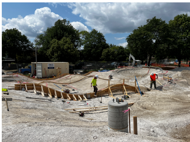
Pump Track Progress – Site
