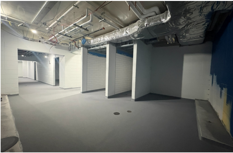
Epoxy Flooring in Showers
