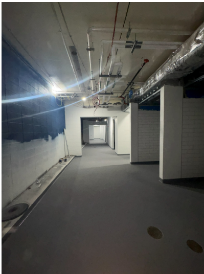
Epoxy Flooring in Locker Room
