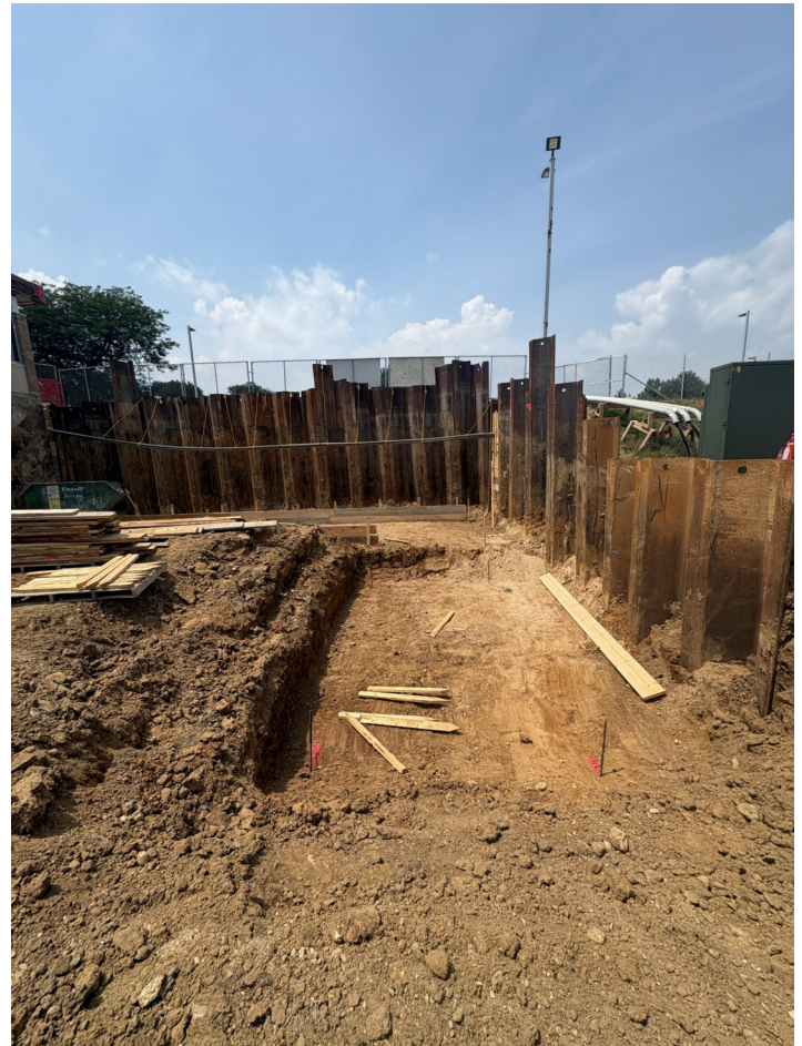
Sheeting Piling for new Gym
