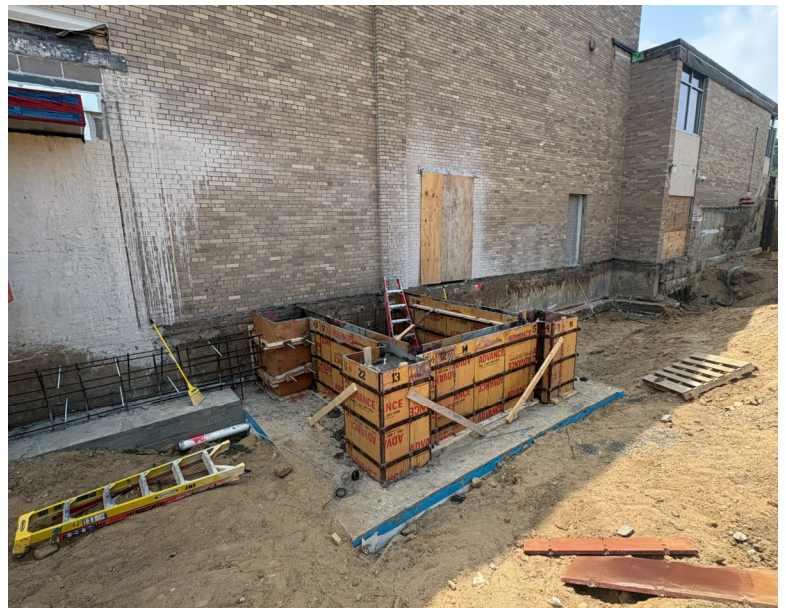
Gym Addition Elevator Pit
