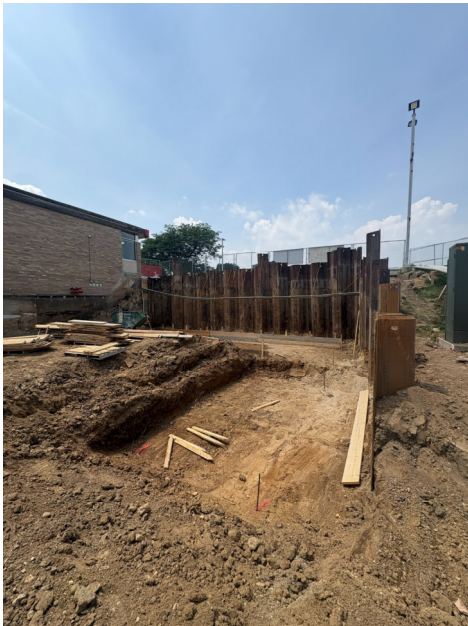
Concrete Footing next to Sheet piling
