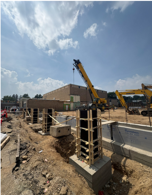
Gym Foundation Work
