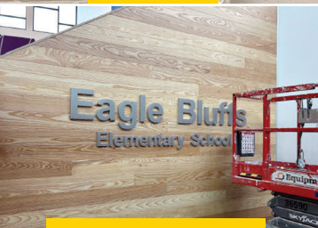
Eagle Bluffs Elementary School Progress
