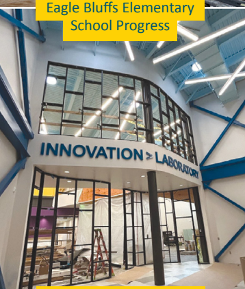
Eagle Bluffs Elementary School Progress
