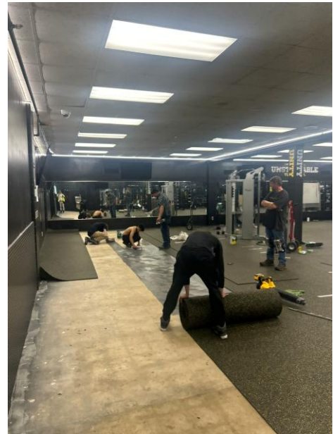
Weight Room Flooring Install
