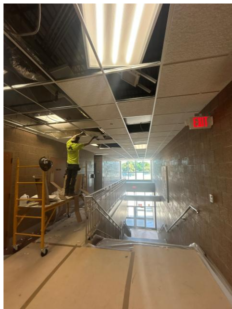
Area E - Stairwell Pad Out
