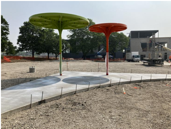
Concrete Poured – Sports Court
