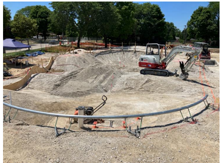
Concrete Forming – Pump Track
