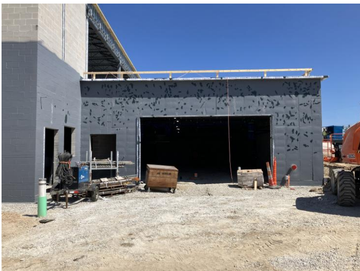
Water Proofing – Area B1 South Side
