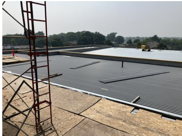
Roof Decking – Area B
