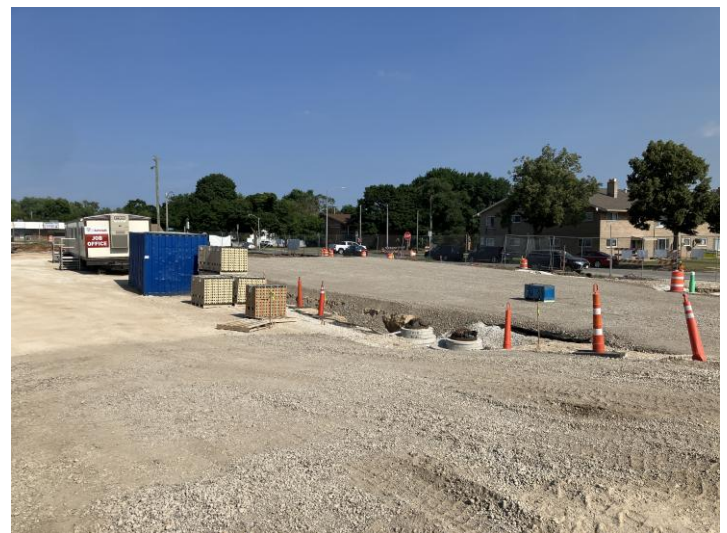
Site Grading – South Parking lot
