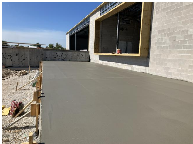
Concrete Topping Poured – Area B1 East Side
