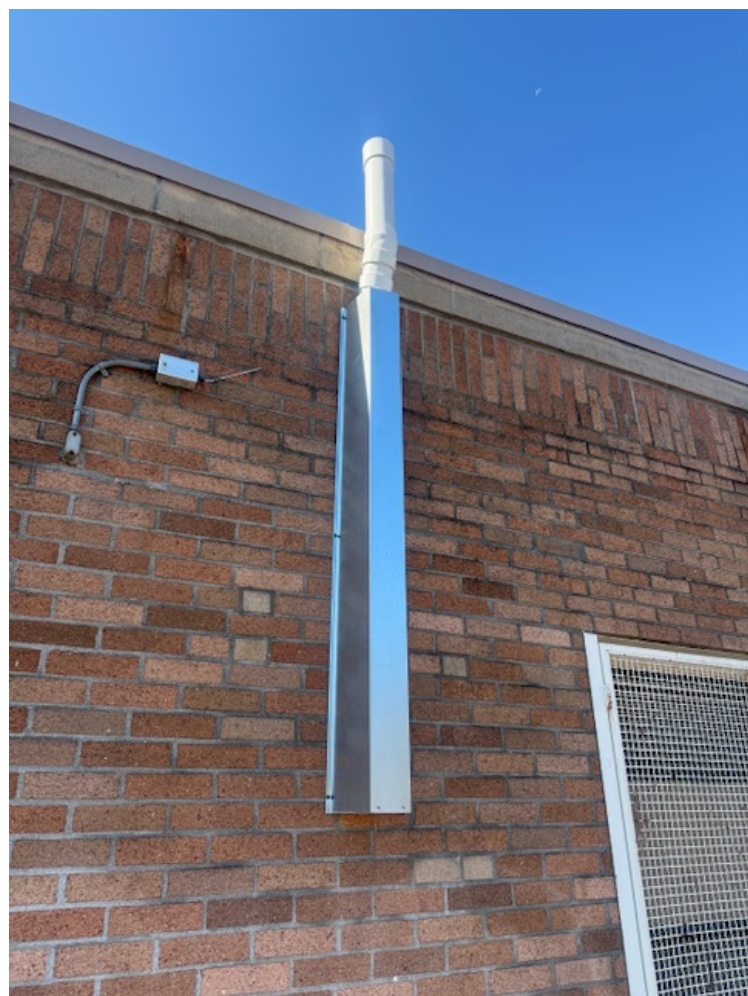
A pipe shroud was installed to deter climbing.
