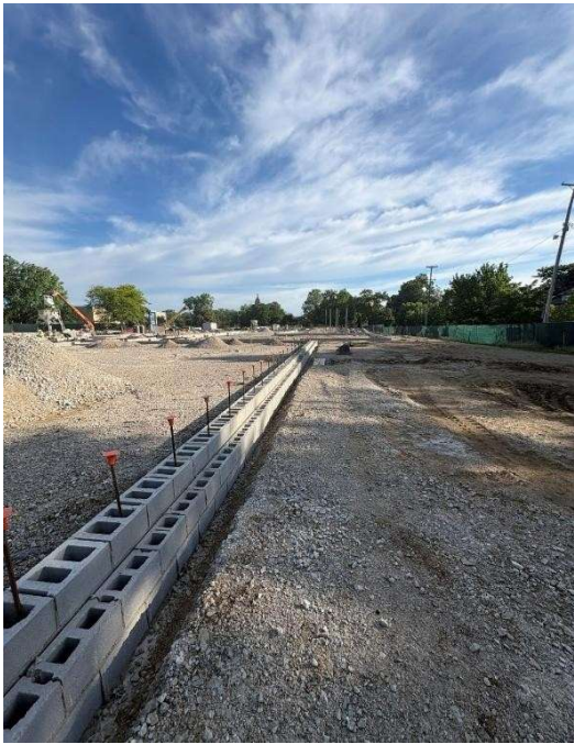
Foundation Masonry at the East Gymnasium Wall
