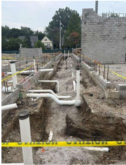
Underground Plumbing, Corridor 1C1
