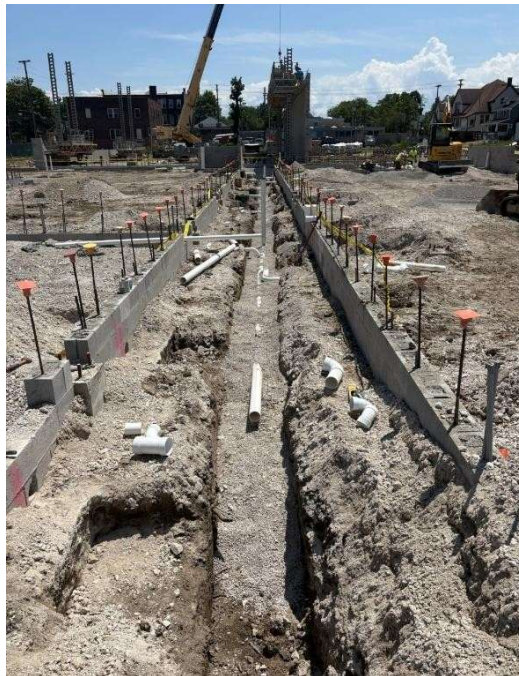
Underground Plumbing, Corridor 1C8
