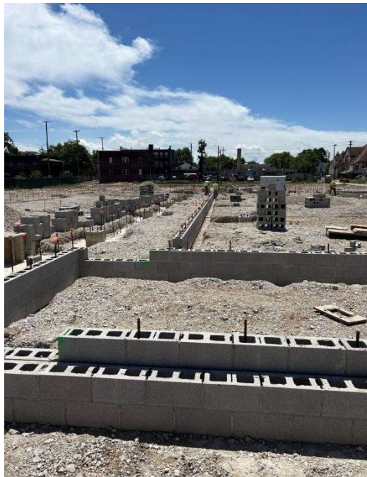
Southwest Foundation Masonry, Corridor 1C7
