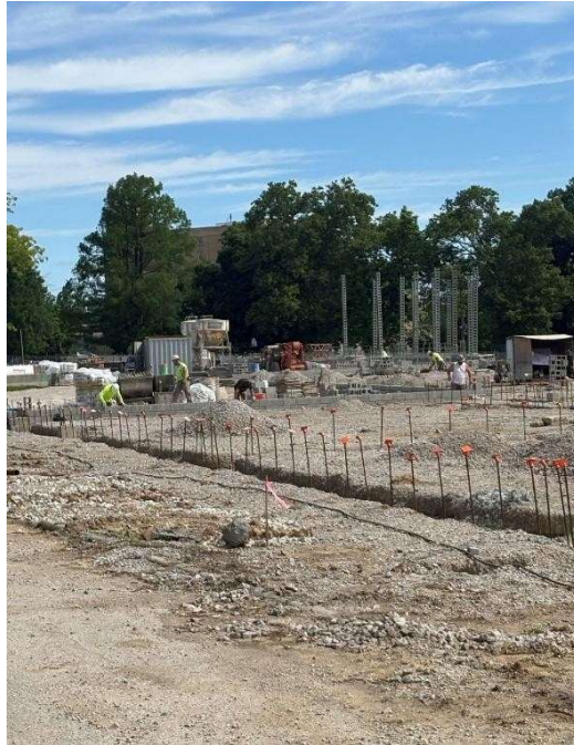
Start of Foundation Masonry at the North End
