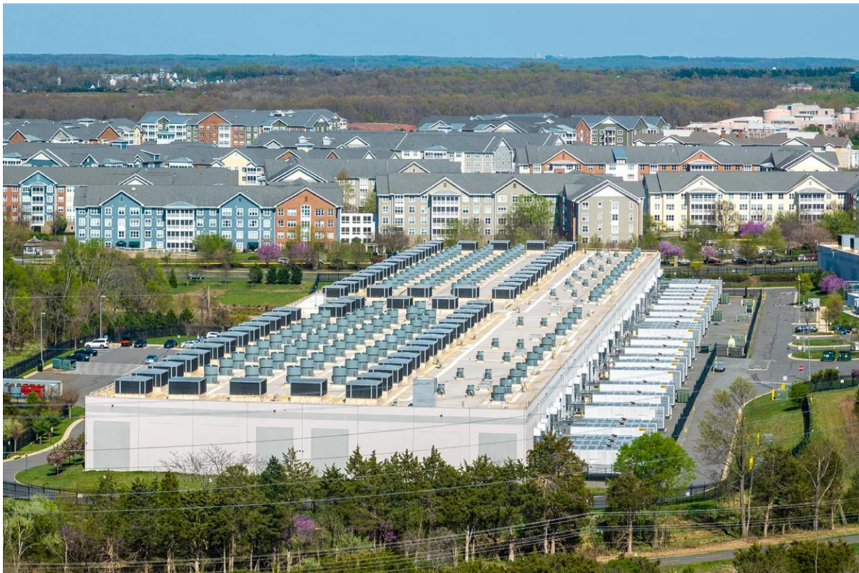
Data Center in Ashburn, VA. Photo credit: Hugh Kenny, Piedmont Environmental Council
