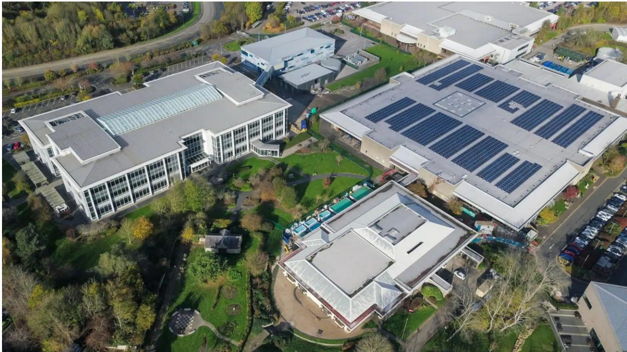
A colocation data center. Image credit: Hanwah Data Centers, reproduced through Creative Commons license CC BY-NC 4.0 ( https://creativecommons.org/licenses/by-nc/4.0/ )
