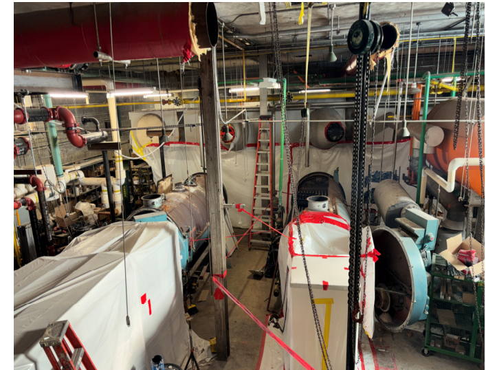
MS Boiler Room Demo
