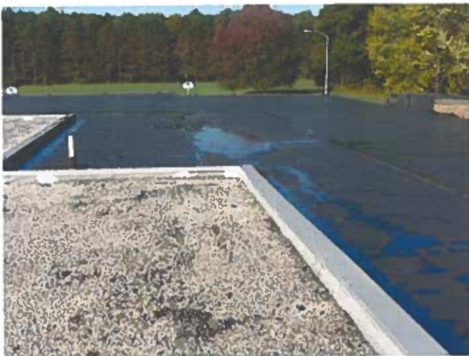
Existing EPDM Roofing
