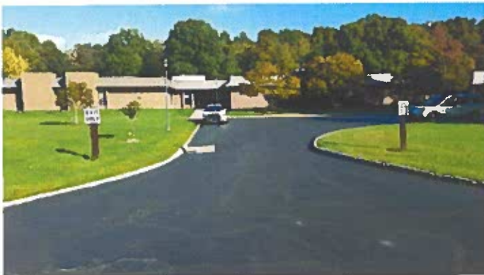
Typical Pavement Condition
