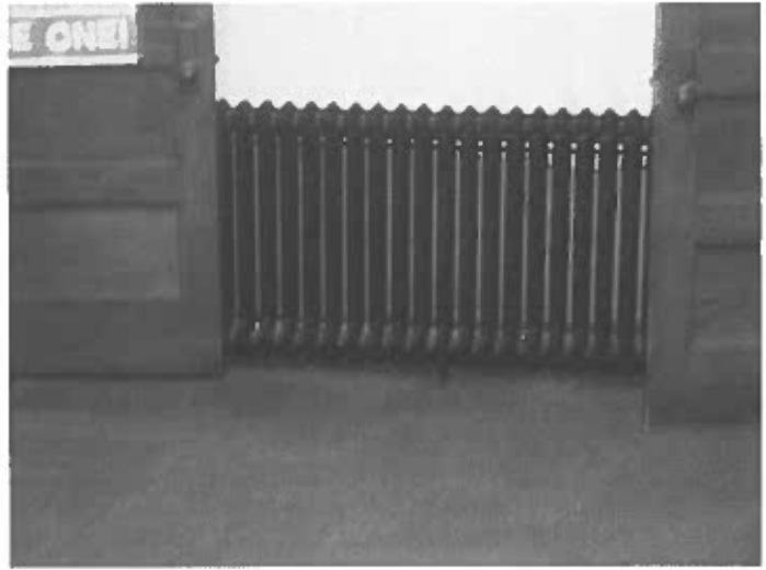
Steam cast iron radiator
