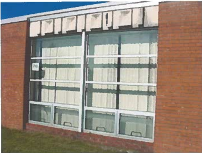
Typical Classroom Window
