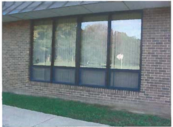
Typical Exterior Window
