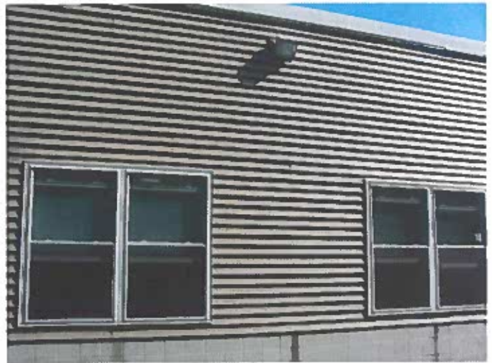
Typical Classroom Windows
