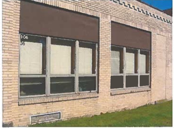
Typical Classroom Windows
