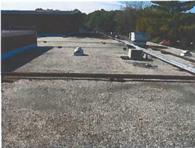
Typical Roof Membrane
