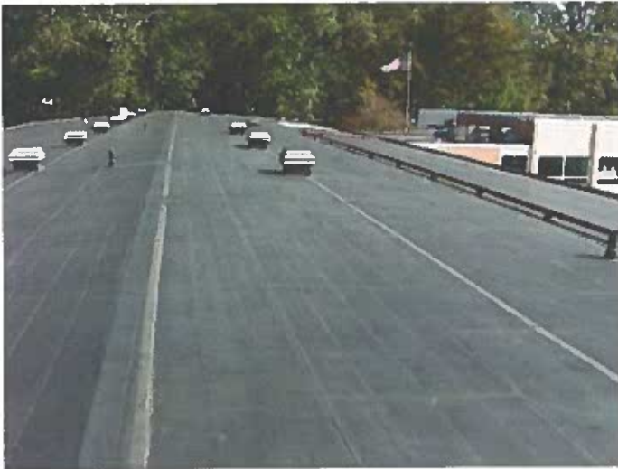
Existing EPDM Roofing
