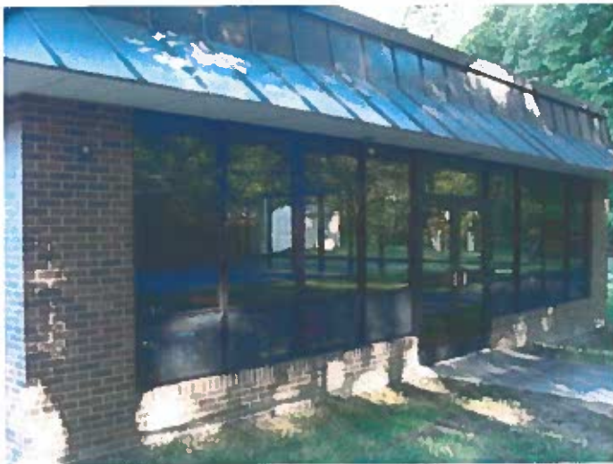
East End Cafeteria Windows
