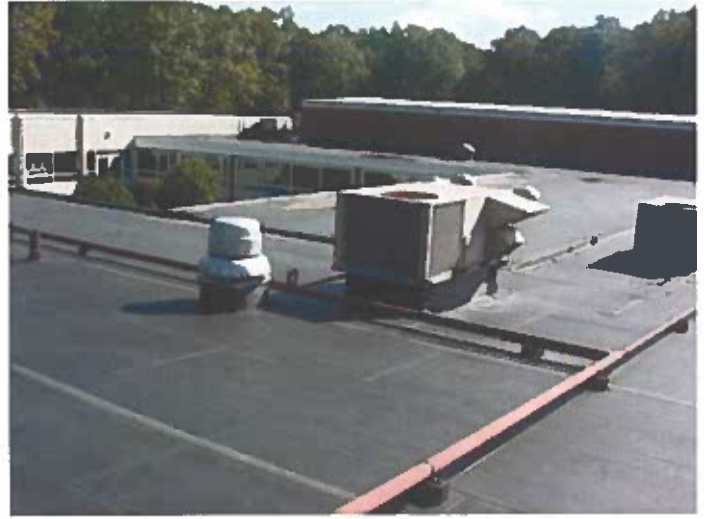
Existing EPDM Roofing
