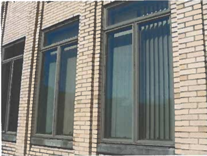
Typical Classroom Window
