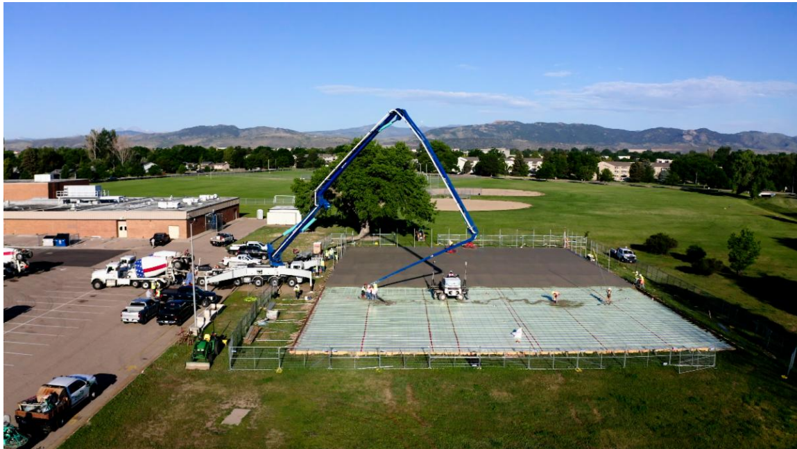
Mill Levy funds are being put to good use— so much is being built and fixed around the district! Photo by Matt Gohl of Boltz's new tennis court
