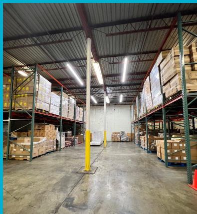
Rack system design and install
