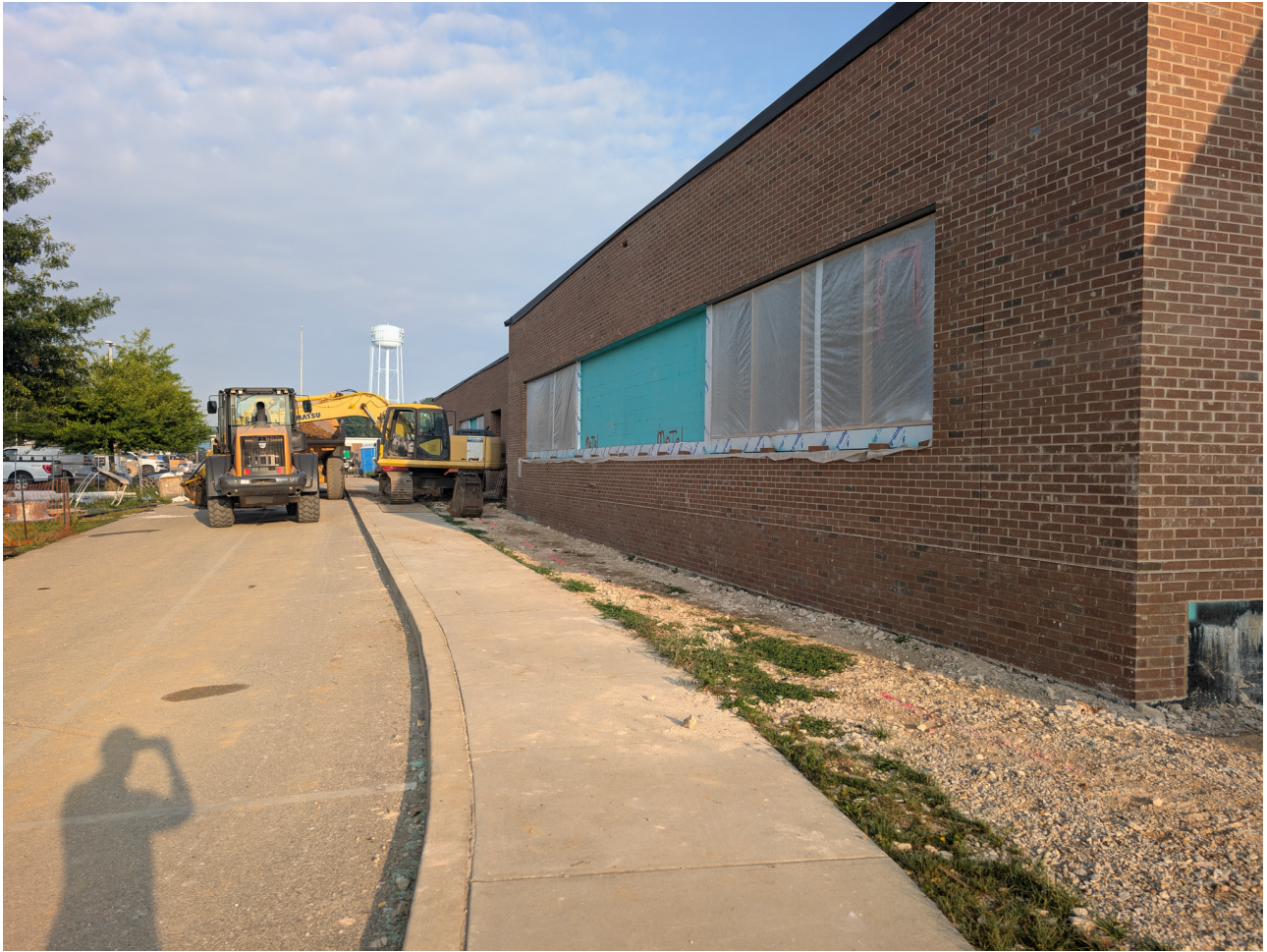
Brick Installation South Wing Area D
