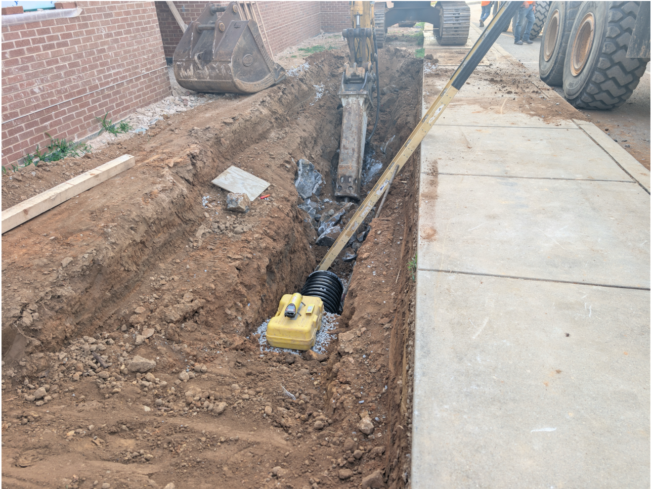
Storm Line Installation Front of Area D
