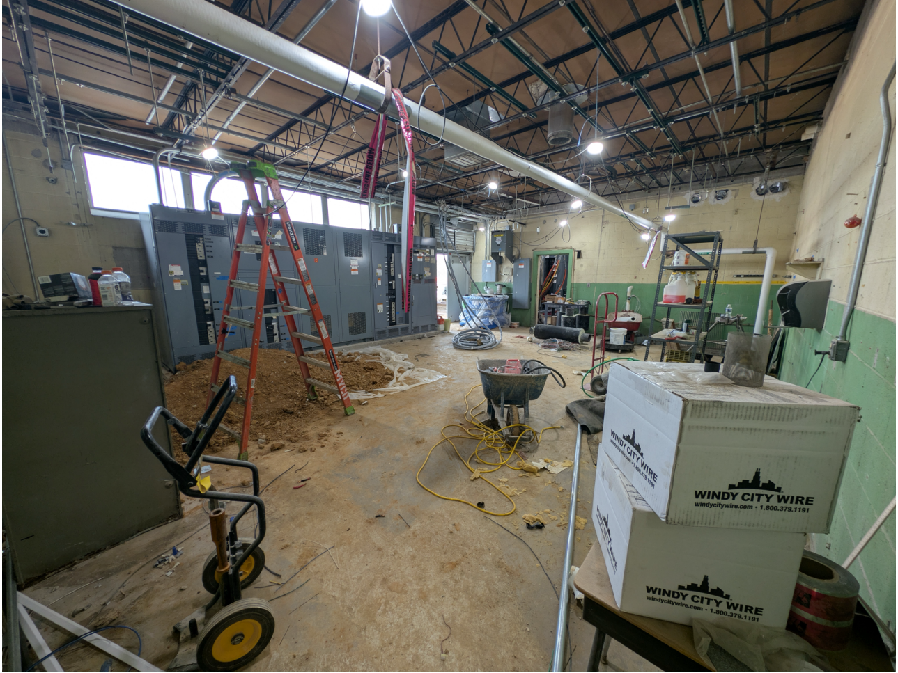
Plan West Mechanical Room Boiler Demolition Complete
