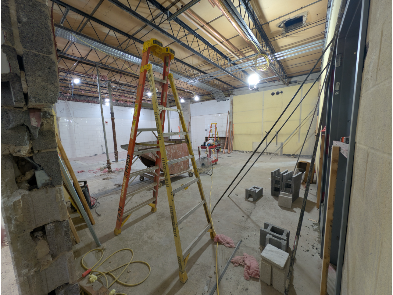
Existing Gang Bathroom Demolition Classroom Wing 1 Area C
