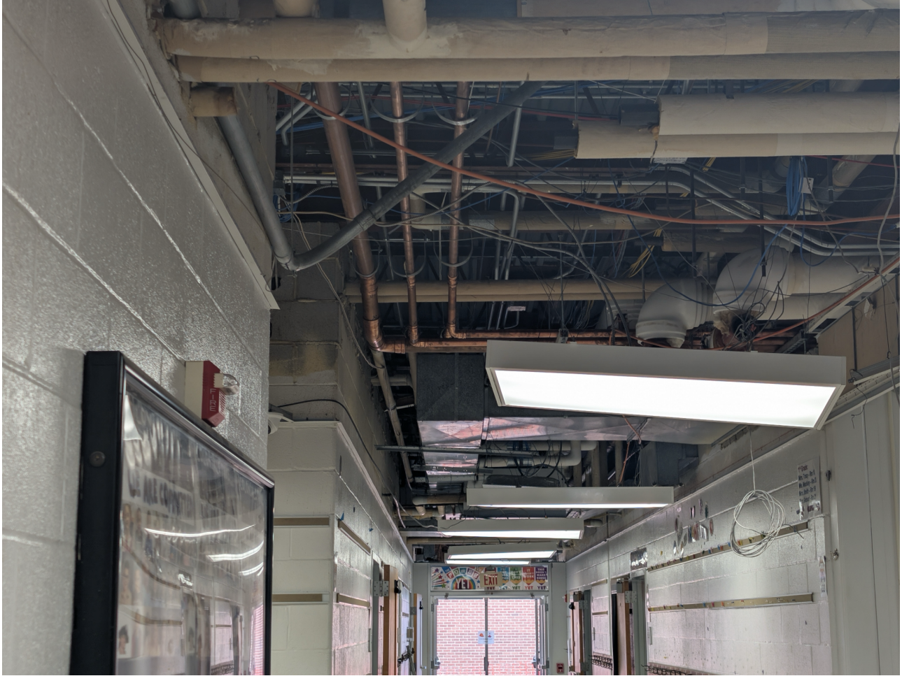
New Copper Water Lines Through Existing Building
