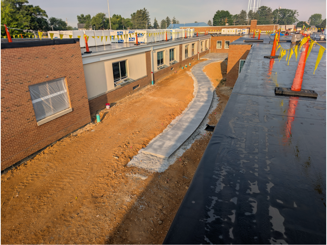
Courtyard Sidewalk Progress Area D
