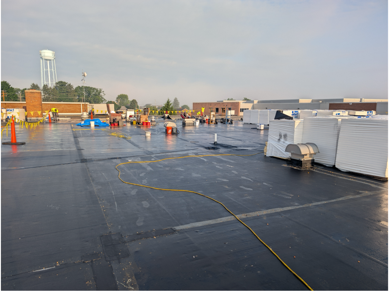
Existing Roof Demo and Install of New Roof
