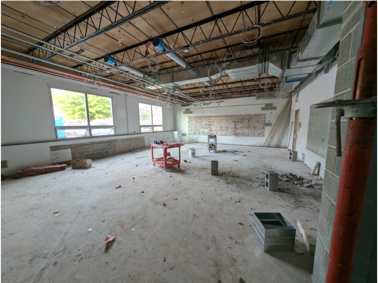
Demolition of Classroom in Classroom Wing 1 Area C
