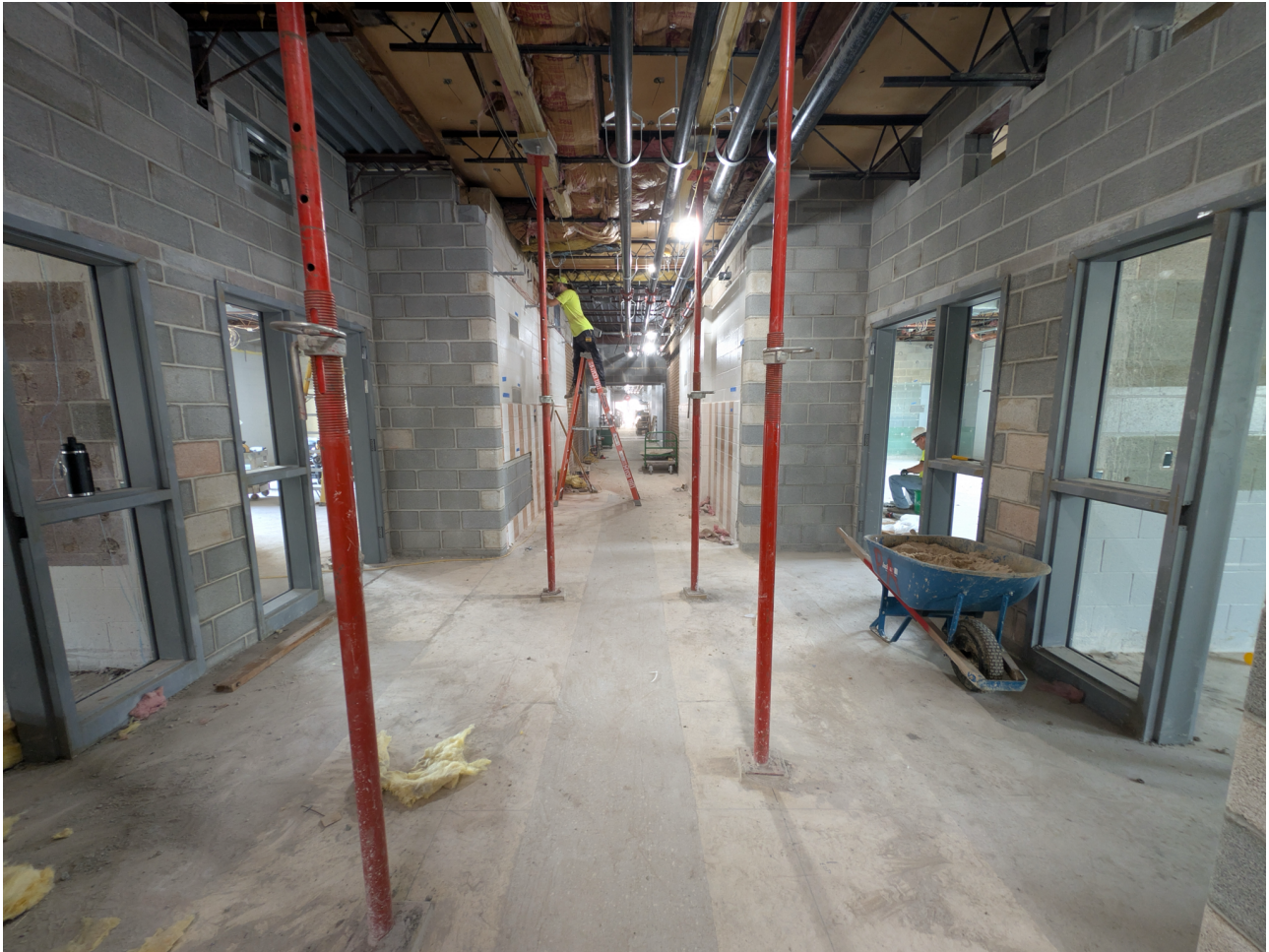
Completed Alcoves Classroom Wing 1 Area C
