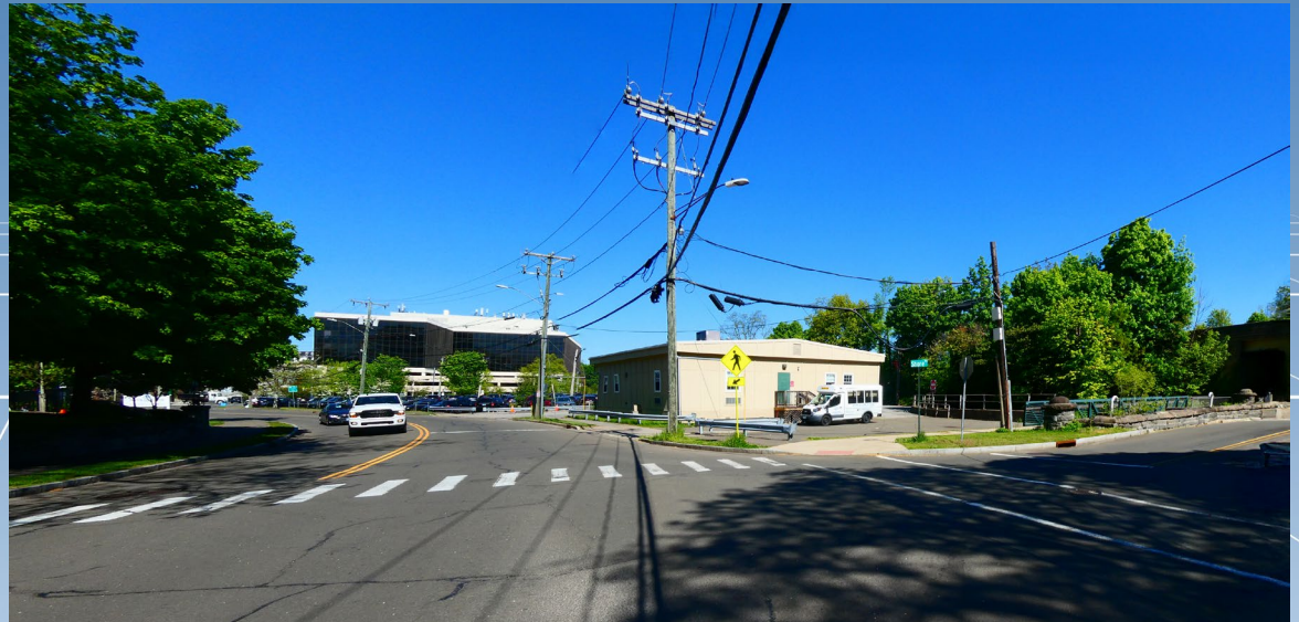
Existing Building and Site – Northwest View
