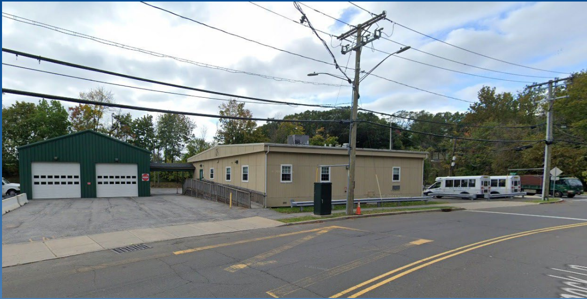
Existing Building and Site – Northeast View
