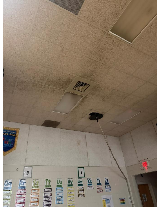
Gym – particulate around ceiling supplies
