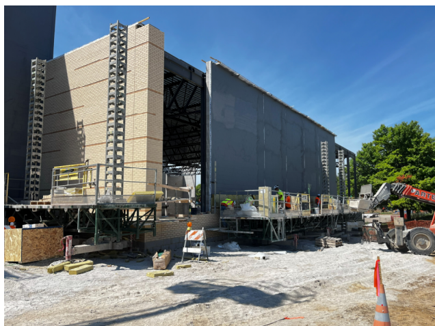
Brick Veneer Progress – Area C2 North Elevation
