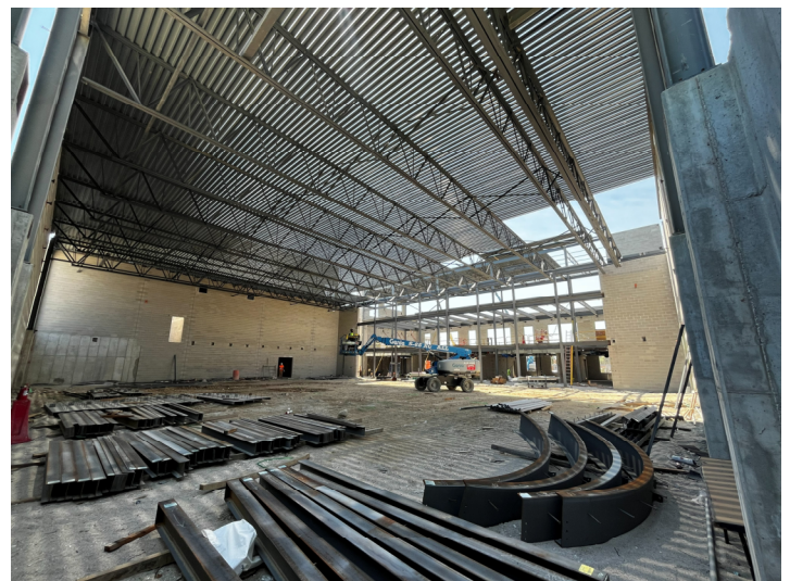
Gymnasium Roof Decking – Area C2
