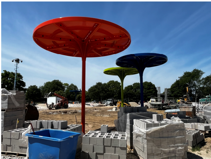
Shade Structures Installed – Site
