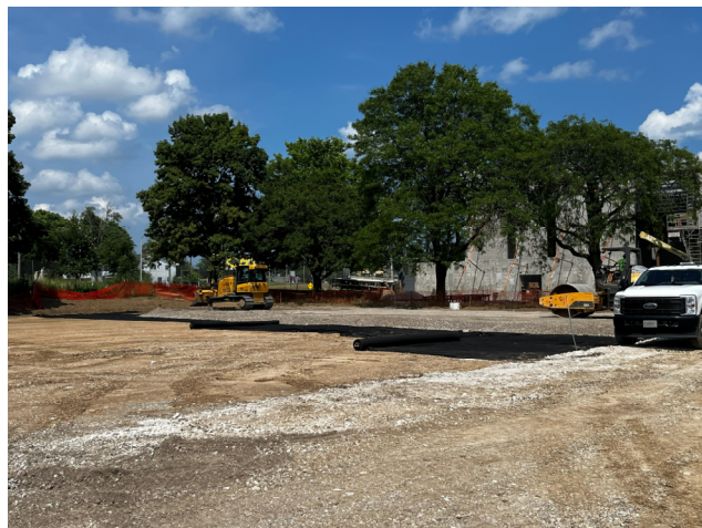
Proof Rolled & Grade – Site - Sport Courts
