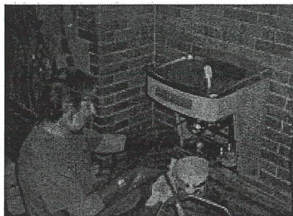
A repair man hard at work on the third floor fountain
