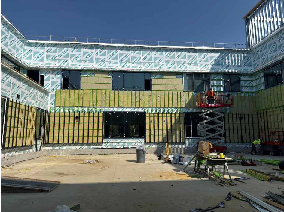
Courtyard progress – AVB, insulation, girls, CMU base.
