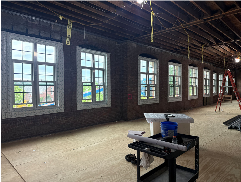
New windows and AVB, Historic Building Level 2.
