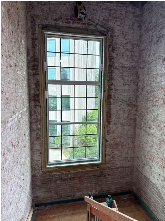
New window at North Stair, Historic Building.
