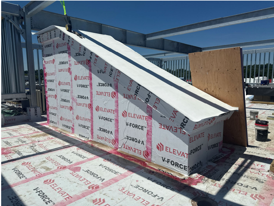
June xx: Waterproofing at roof access stair enclosure
