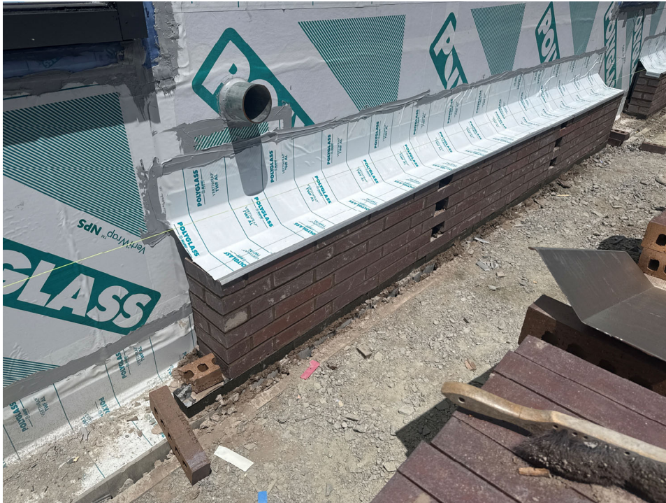
Start of brick and flashing, East elevation.
