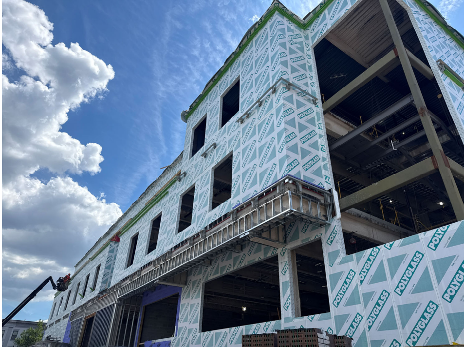
West (School Street) elevation – framing and AVB.
