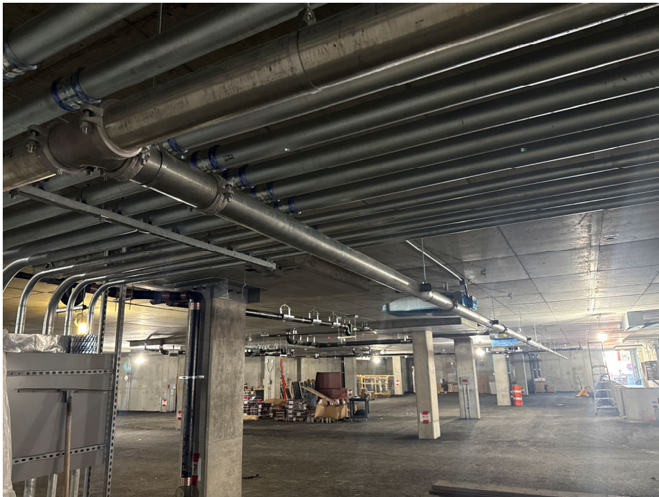
Sprinkler piping installation, garage level.
