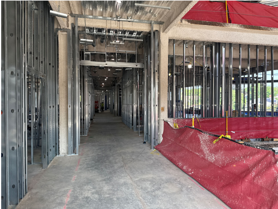
Interior wall framing, Building B level 2.
