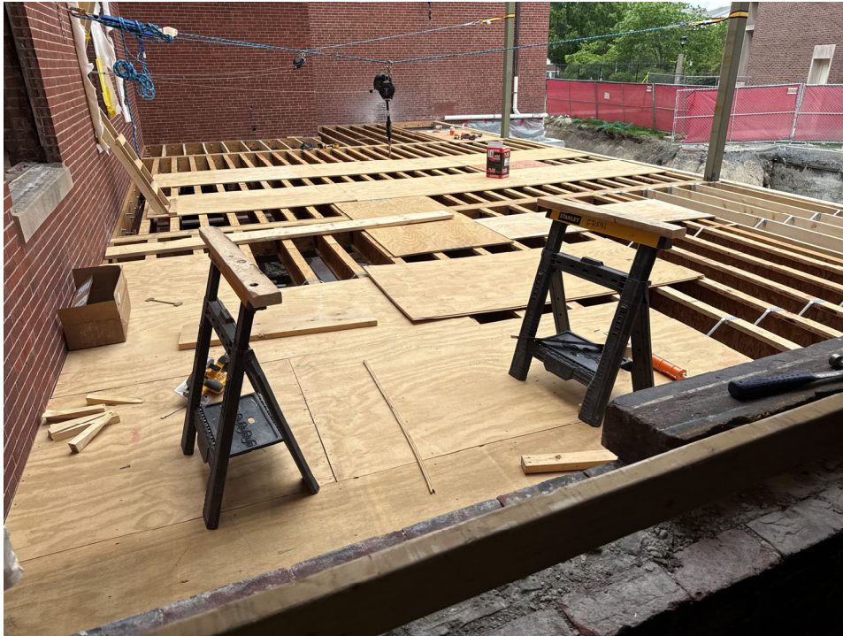
Historic Building Addition – wood framing and decking, L1.
