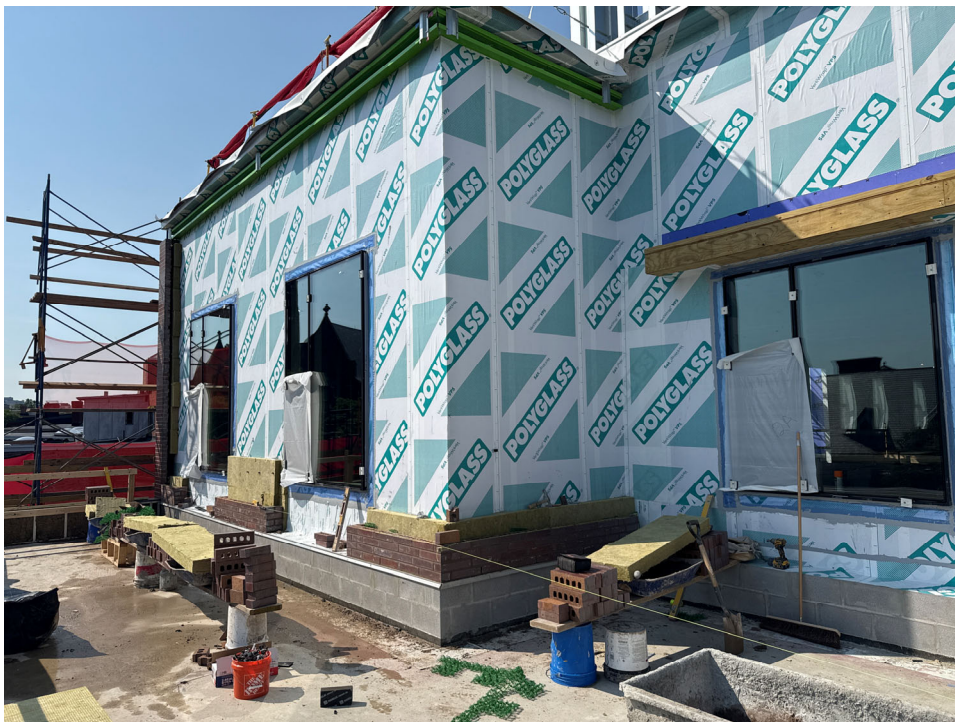
Brick progress, North elevation Building A.
