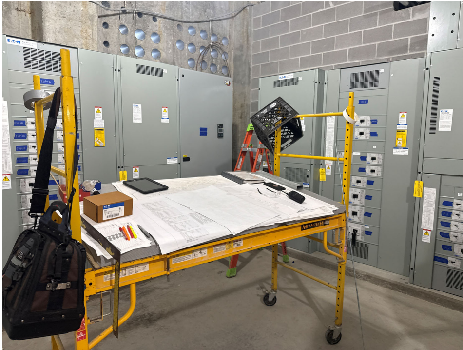
Installation of electrical gear, main electric room B1.
