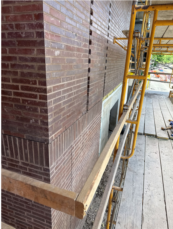
Brick progress, North elevation.
