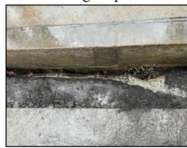
Images showing spalled concrete and exposed rebar at bridge joint on the underside of bridge and along curbline.
