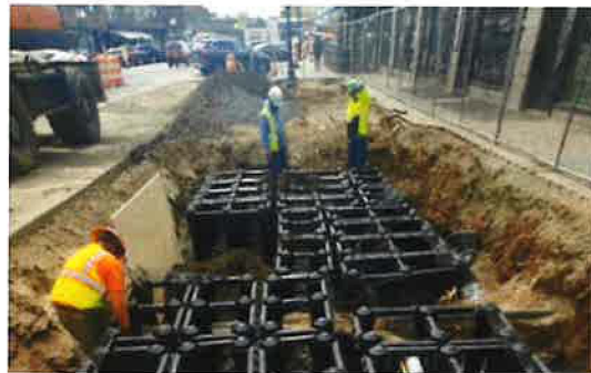
Tree Soil Cells on LaSalle Road
