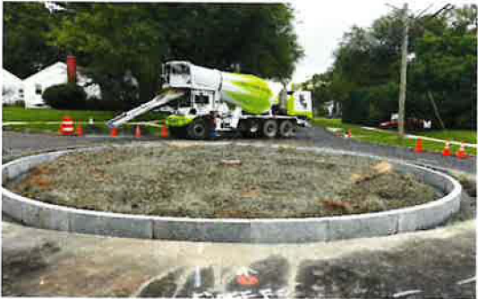
Roundabout Construction on King Philip Drive
