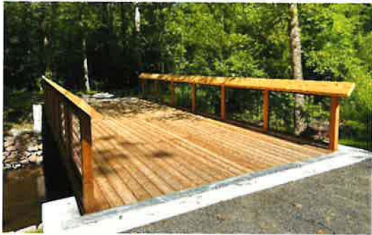
Westmoor Park Pedestrian Bridge Replacement
