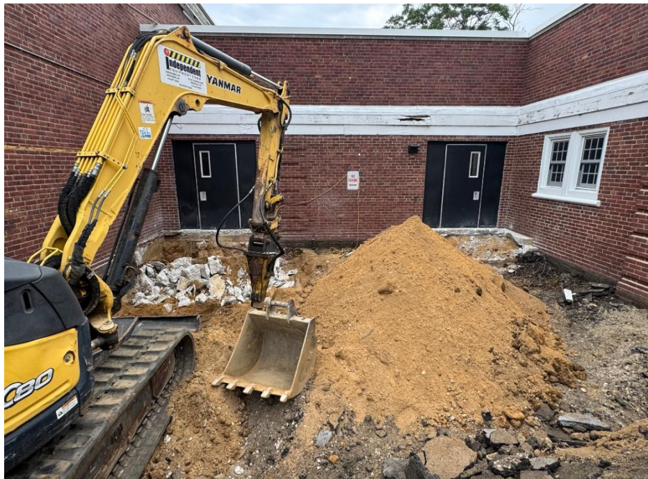
Hempstead McNeil ES – Elevator Excavation
