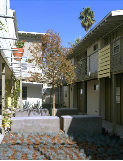
Waterloo Affordable Housing, KoningEizenberg
