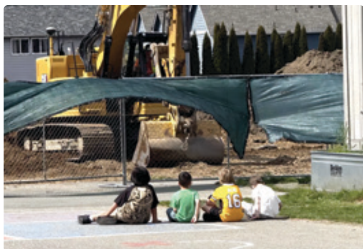
Hillcrest Elementary School students watch the construction of their new gymnasium, which is scheduled for completion in the winter of 2027.
