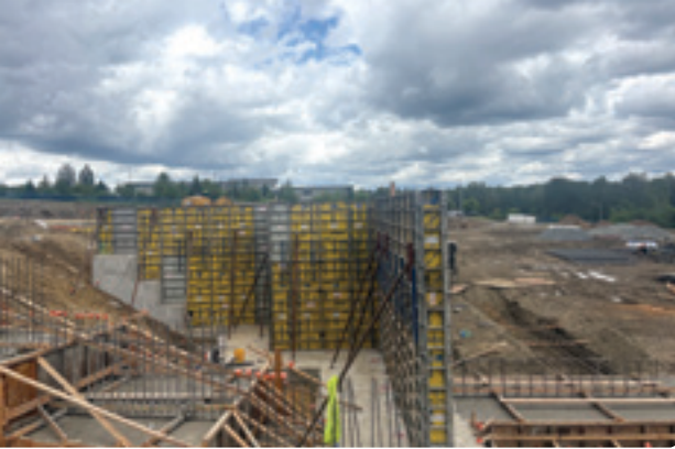
Site preparation and infrastructure work are underway for our eighth elementary school. Once complete it will serve Glenwood Elementary School students and staff, followed by Lake Stevens Middle School students and staff.
