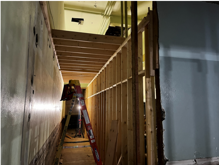
Wood Framing – Area A1 1 st Floor
