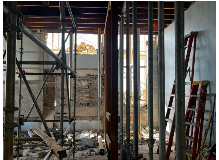
Demolition – Area A1 3 rd Floor
