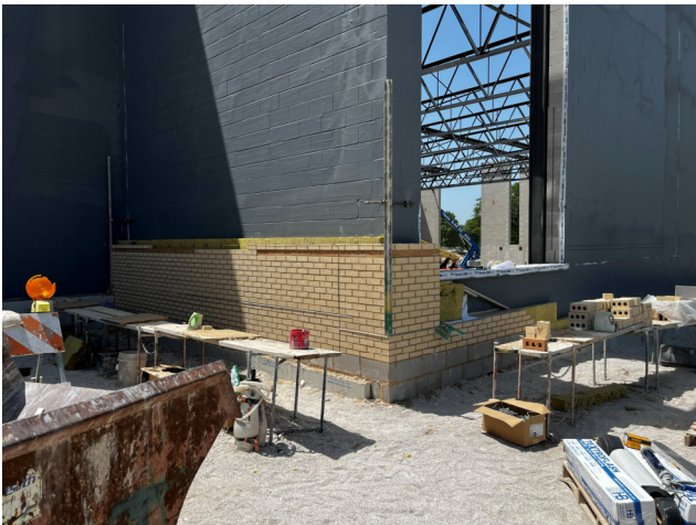
Brick Veneer Started – North Elevation
