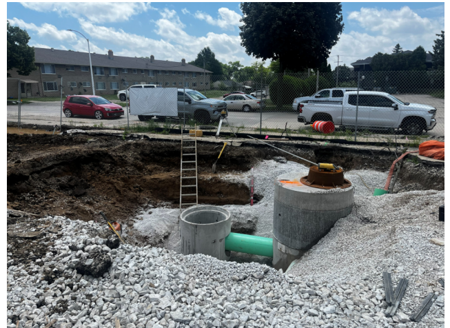
Storm Drain Installed
