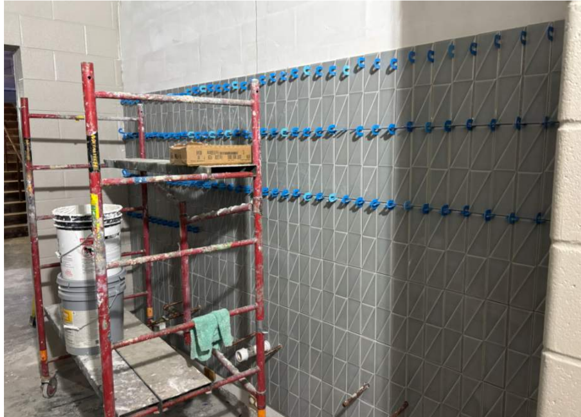
Bathroom Wet Wall Tiling – 5/19/25
