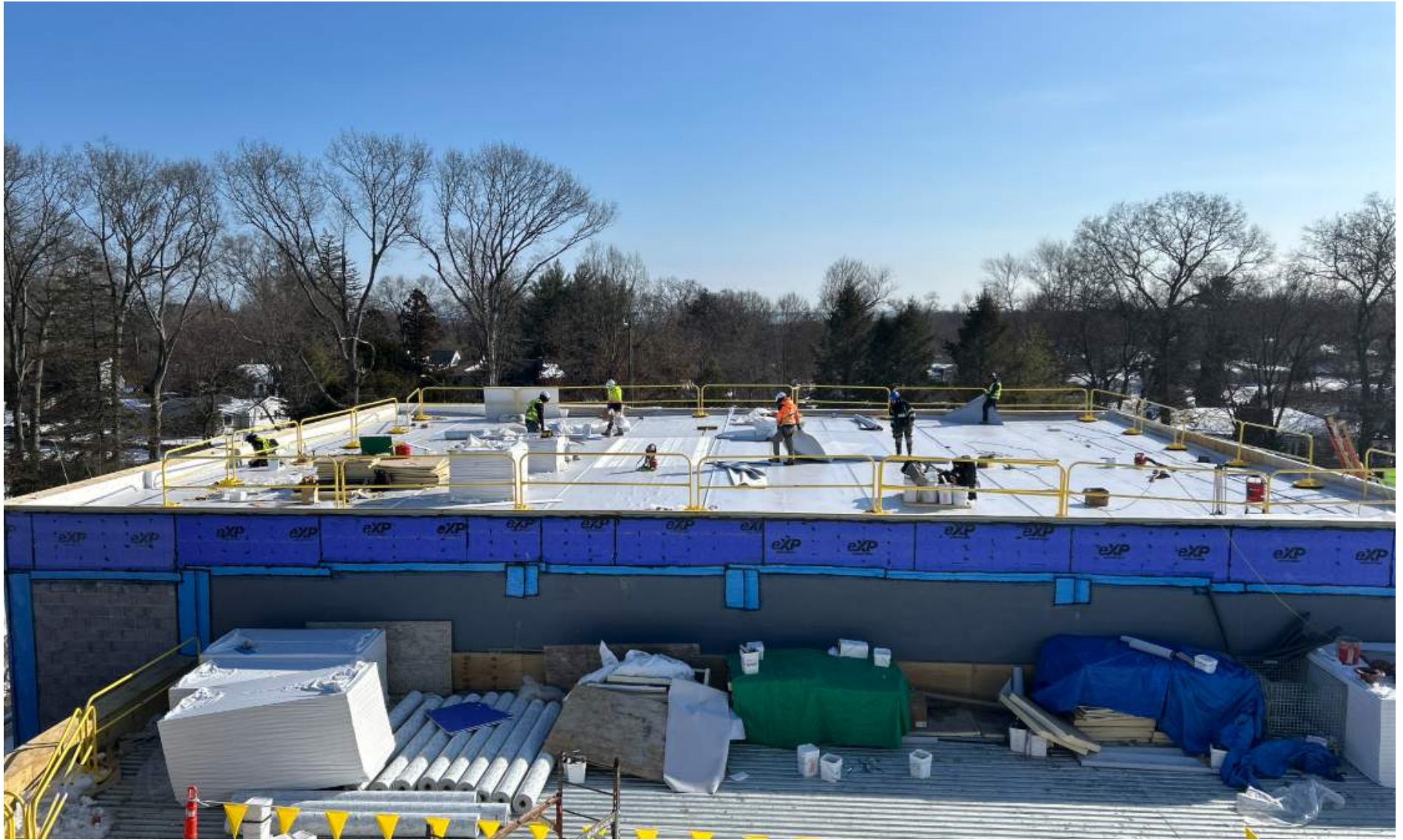
Building Envelope – Ongoing Roofing at Auditorium 2/16/26
