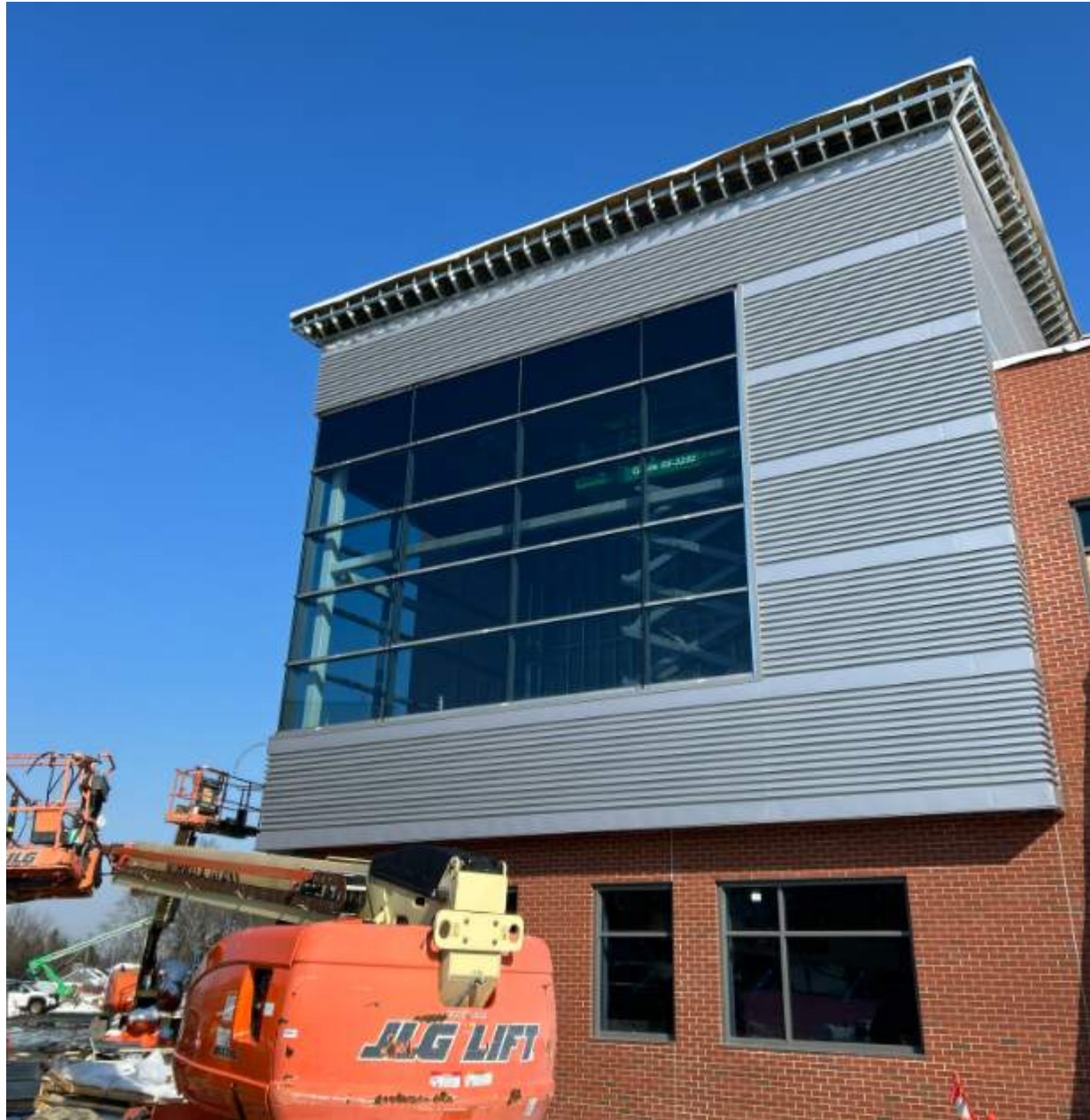
Building Envelope at P-TECH Project Room 2/25/26
