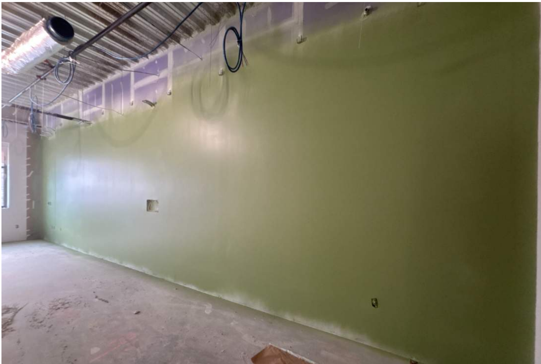
Classroom Finish Paint 1/31/26
