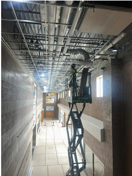
Grid Completion Area F
