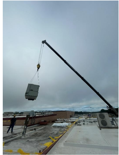
Existing Condenser Removal
