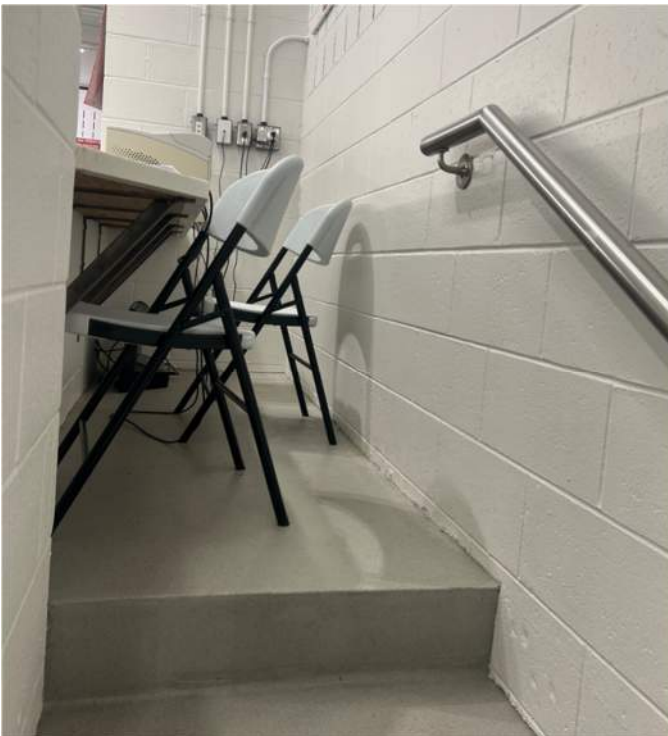
Photo 12: The scorer's platform was constructed as part of the 1997 renovation, on the east side of the pool. It is not handicapped accessible and contributes to the narrow deck along that side of the pool. (See Photo 13)
