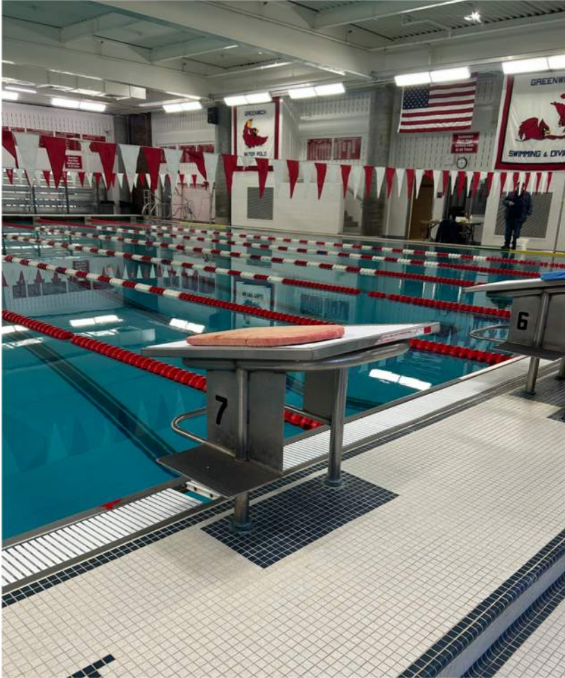
Photo 3 (Left): The Natatorium structure is comprised of structural steel girders, spanning 95-feet, supporting steel beams and deck. The girders are supported by round cast-in-place concrete columns. Perimeter walls are concrete masonry units (CMU) with acoustical CMU in the upper half of the wall. All structural systems appear to be in good condition. Refer to Appendix 1 for Structural Engineer's Assessment.
