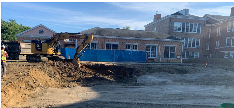
Footprint for new addition nearing completion
