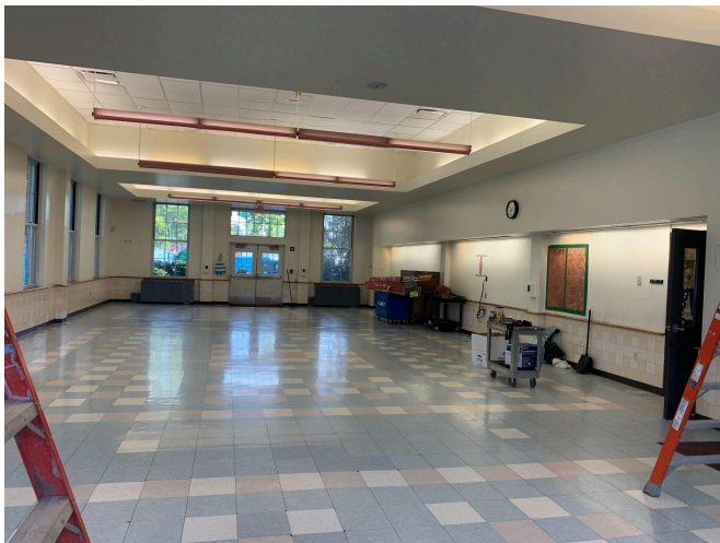
Cafeteria move completed in preparation for renovations
