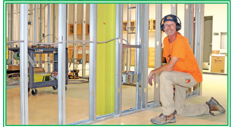
Joe Ludwig of Pearson Construction works on one of two offices being created for the Technology Department at the Central Office. Ludwig is a 1985 graduate of Berrien Springs High School.
