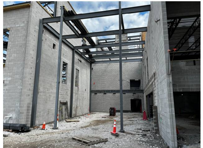
Structural Steel Installed – Area B1 - Main Entrance
