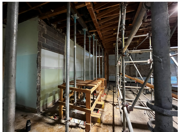
Removed Wood Bearings – Area A1
