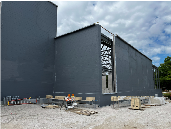
Waterproofing – Area C2 & A2 - North & East Wall
