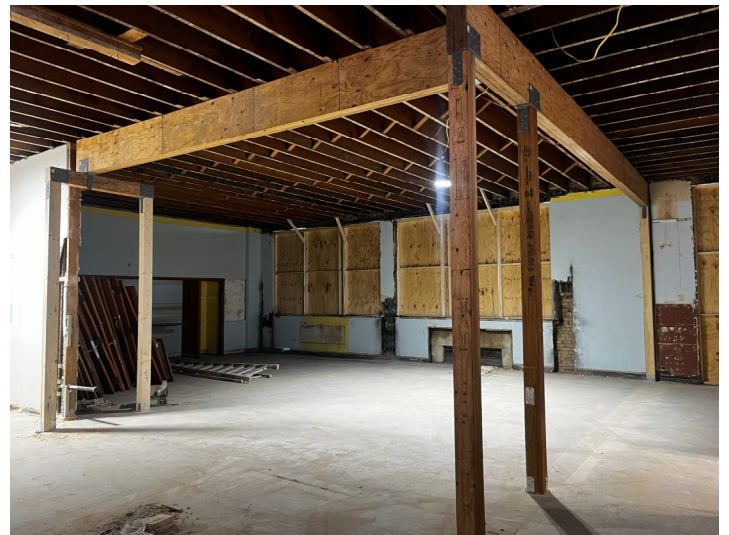
Wood Bearing Framing – Area A1 – 3 rd Floor
