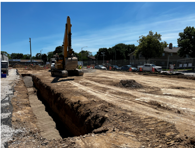
Grading & Storm Drain – Southeast Of Site
