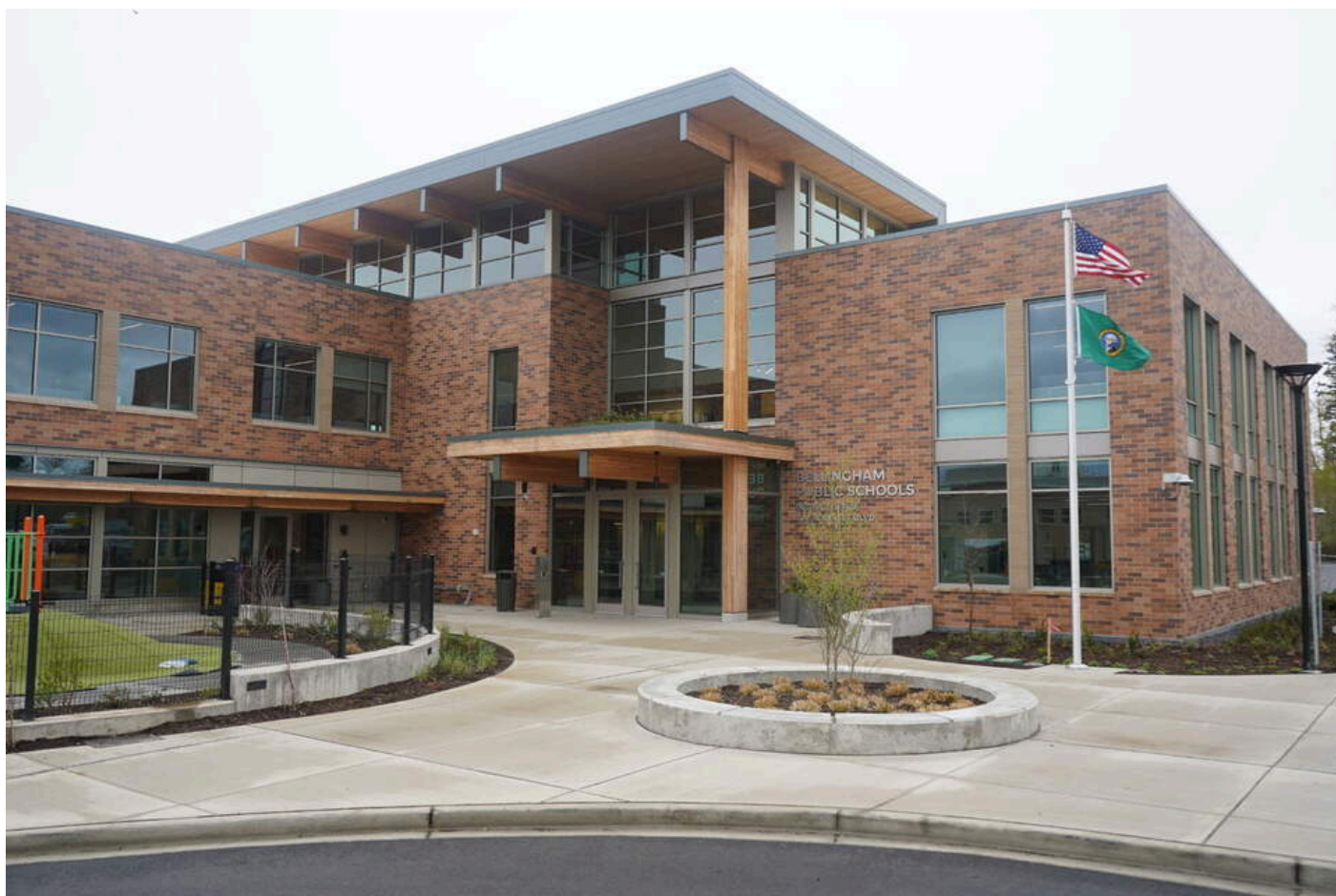
Bellingham Public Schools District Office at 1985 Barkley Blvd. Rachel Showalter The Bellingham Herald
