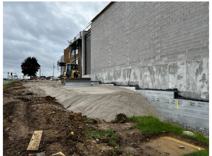
Grading – Northside of Area C2
