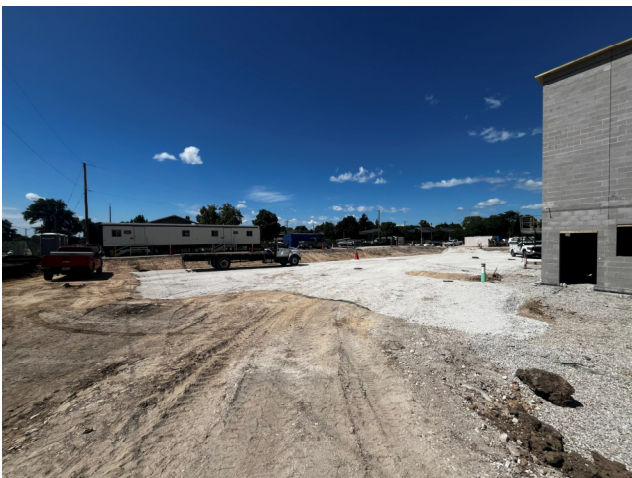
Grading – Southeast Of Site
