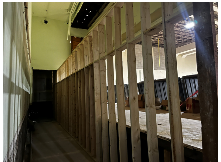
Wood Framing – Area A1
