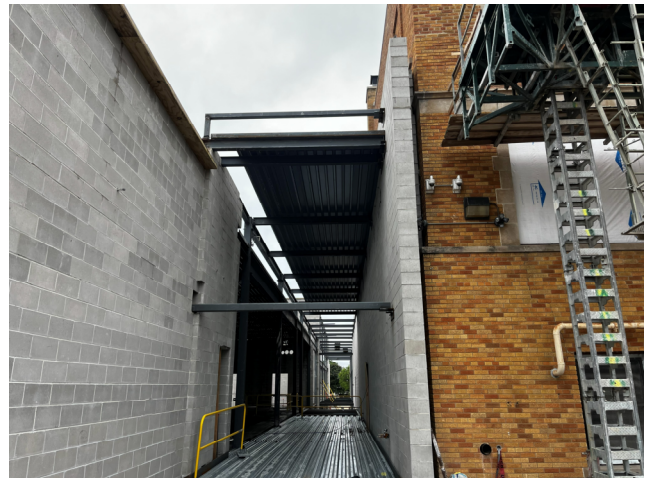
Roof Decking – Area B1
