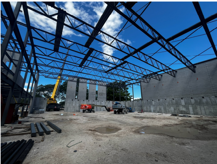
Structural Steel Joists – Area C2
