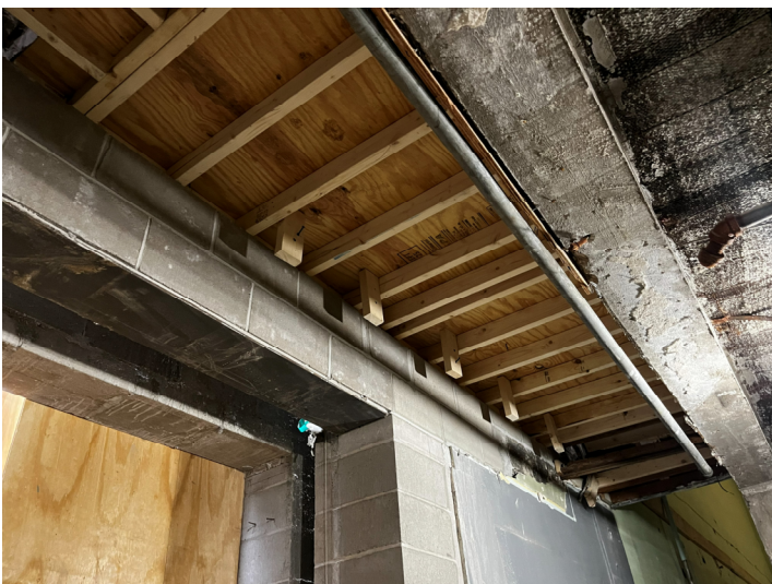
Wood Framing – Area A1
