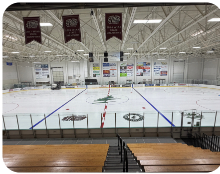
Ice Maintenance Complete
