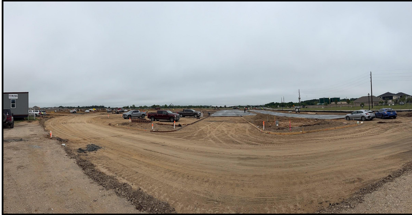
North Parking Lot (first concrete pour)
