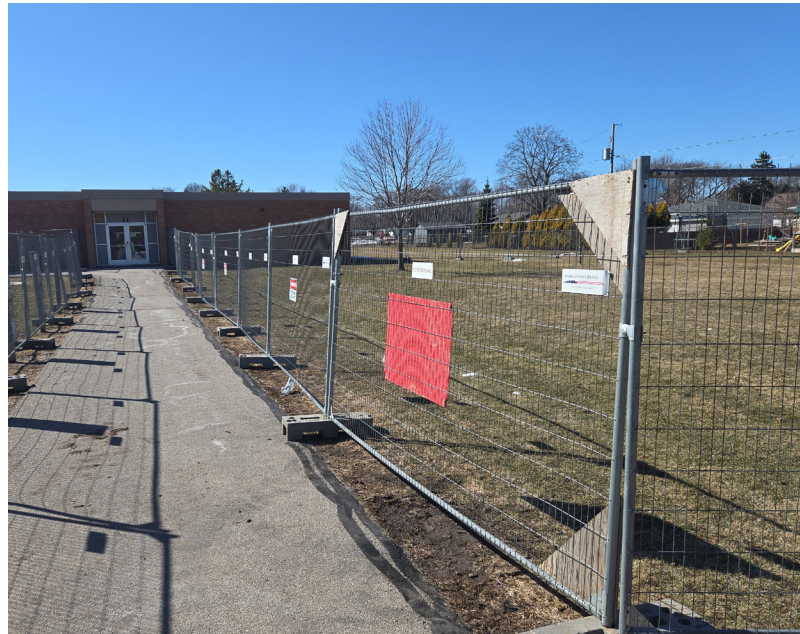
Fencing Installation at Franklin Elementary School
