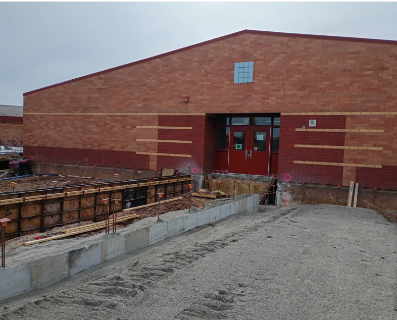
Footing Installation at Carl Traeger Elementary School
