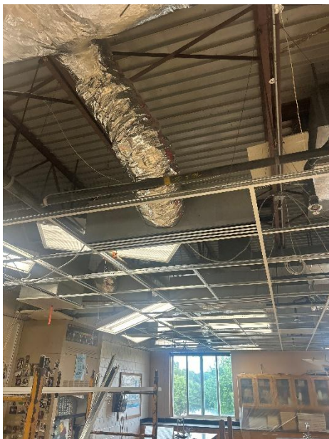
Grid Install Science Room 2018
