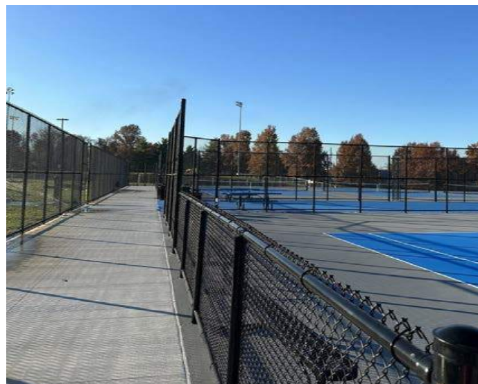
East Concourse Looking South
