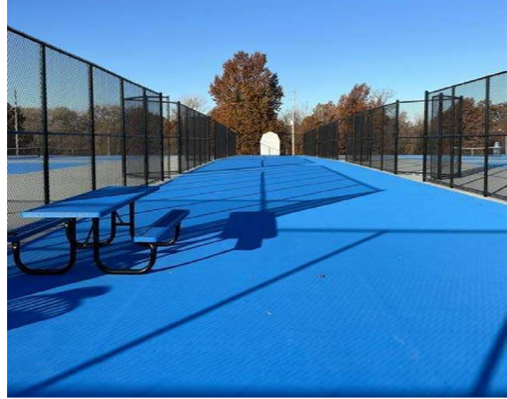
Center Spectator Concourse Looking West
