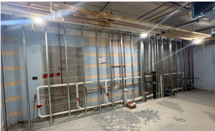
Above: Framing and Inwall MEPF Piping Below: Bus Barn Demo
