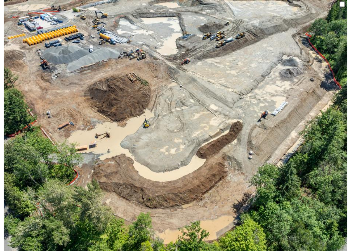
The NW corner of the site showing the stockpiling of dirt in preparation for the installation of retaining walls
