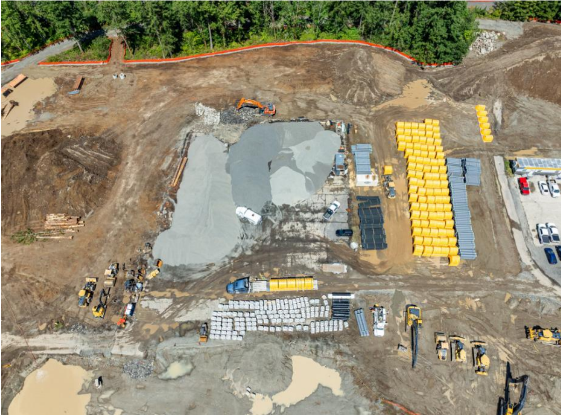
Stockpiling of materials including parts of the underground storm water storage system (yellow)
