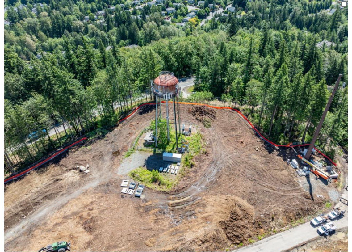
The area around the old water tower being prepped and graded. Water tower is expected to come down in mid-July
