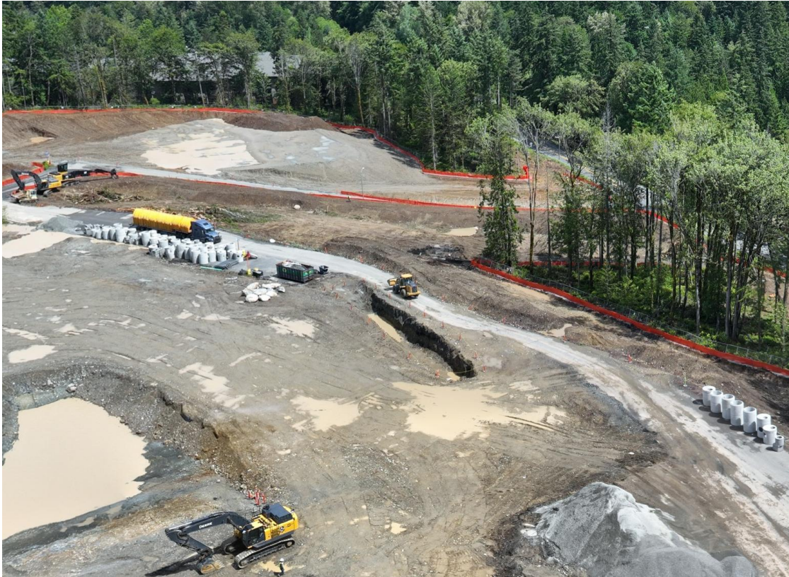
The area of the new entrance drive being graded
