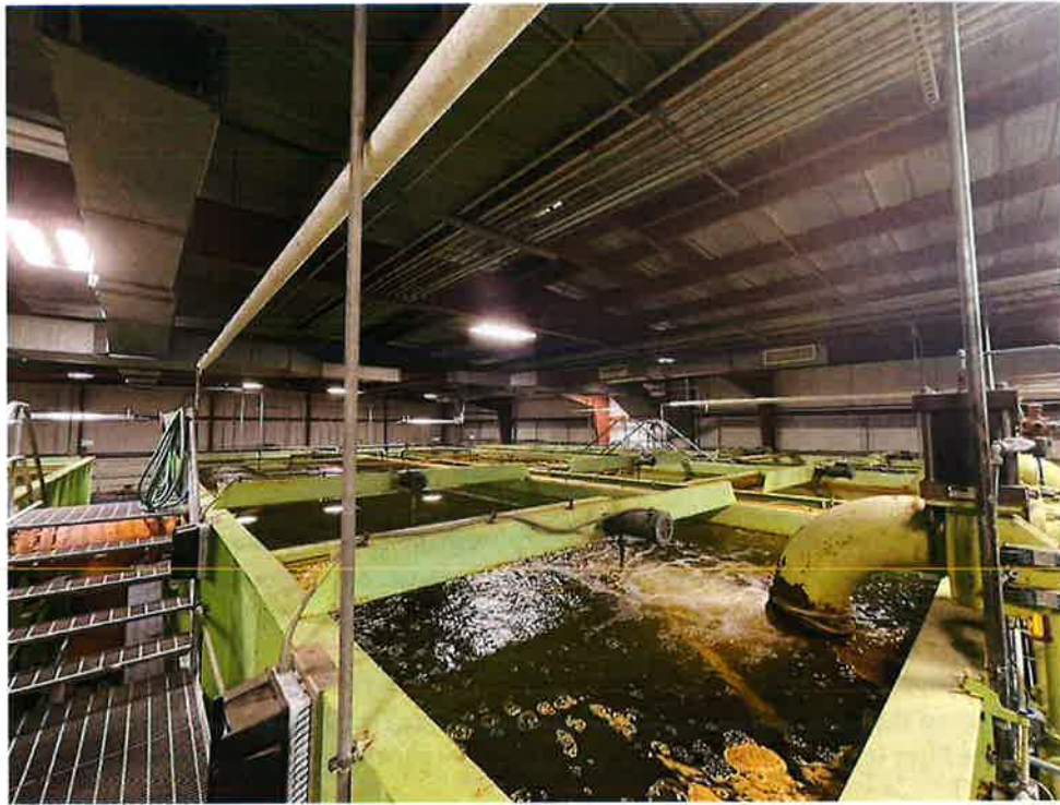
Figure C9. Units 2, 3, and 4 overview.
