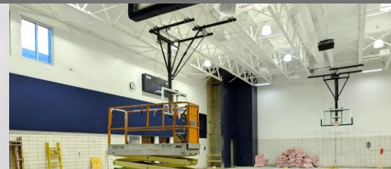
New windows light up the main gym
