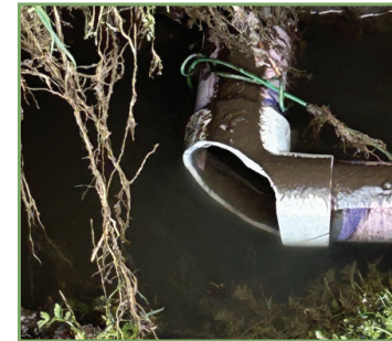
Broken underground water pipe and flooding at Carmelo Child Development Center.
