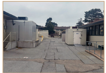
Inadequate space for semi-truck delivery, food storage, and packout deliveries to all other sites from our Central Kitchen at Carmel High School
