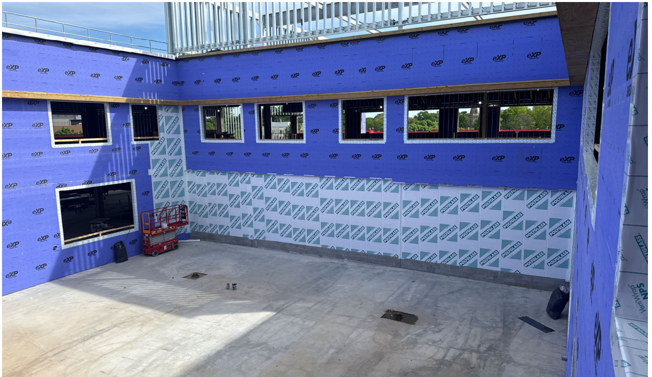
May 26: AVB Installation in Courtyard
