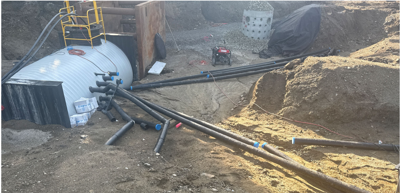
May 20: Connecting Branch Lines to the Vault
