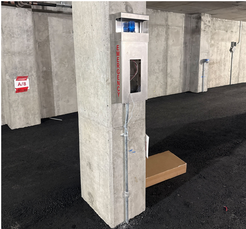
May 14: Emergency Devices Installed in Garage
