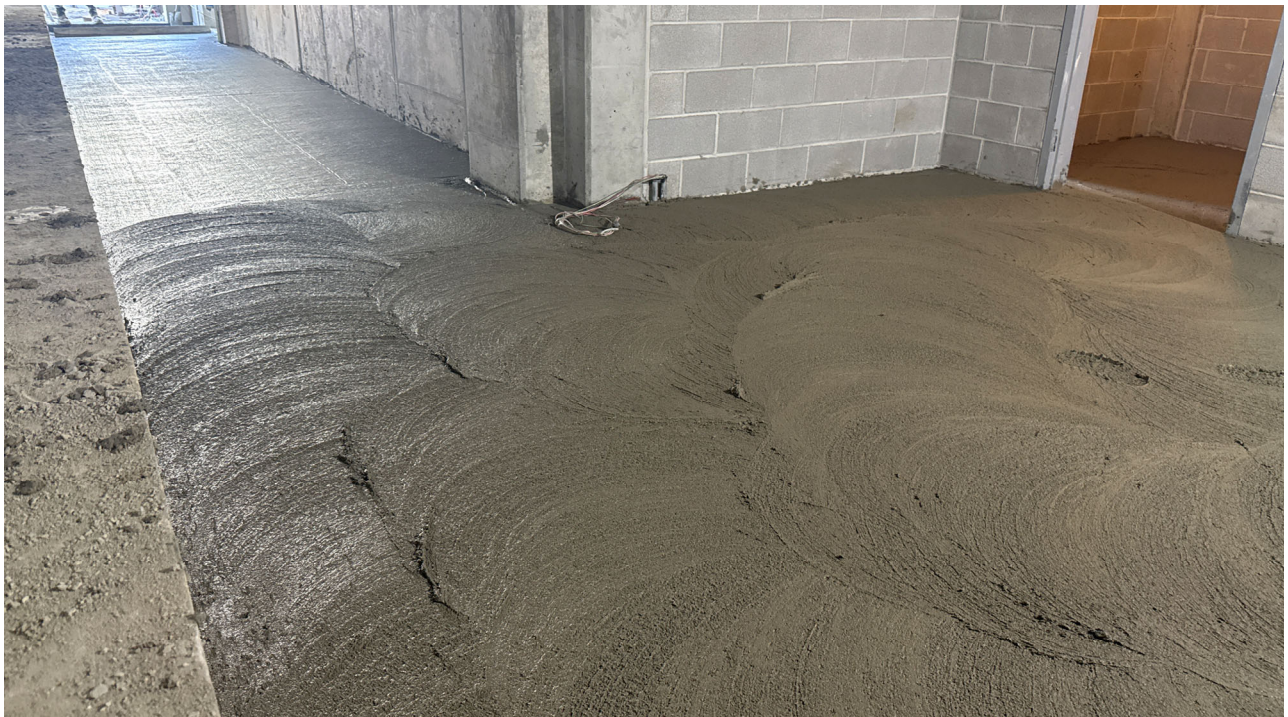
May 14: Concrete Placement at Garage Level
