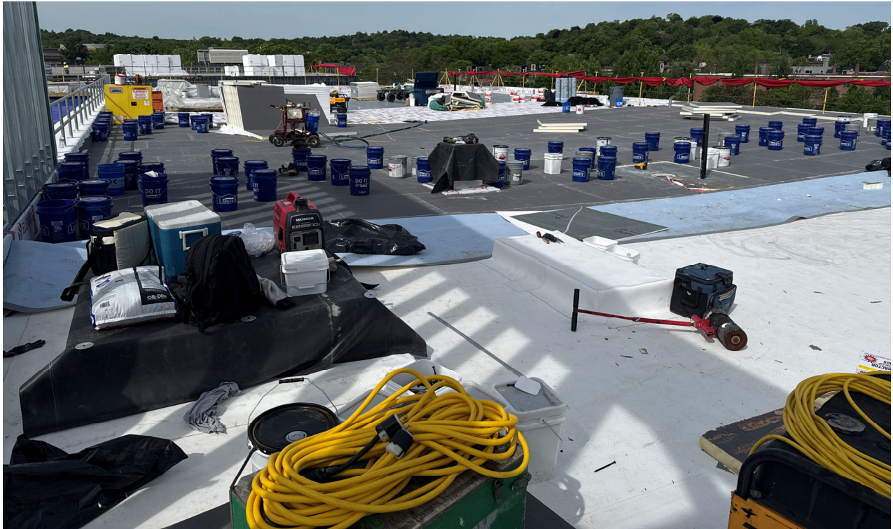
May 26: Roofing progress, Building A West
