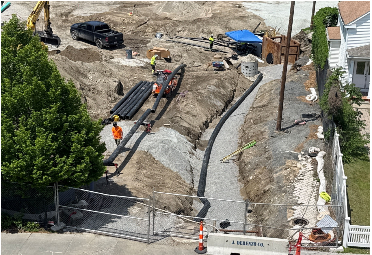
May 20: Geothermal Main Installation
