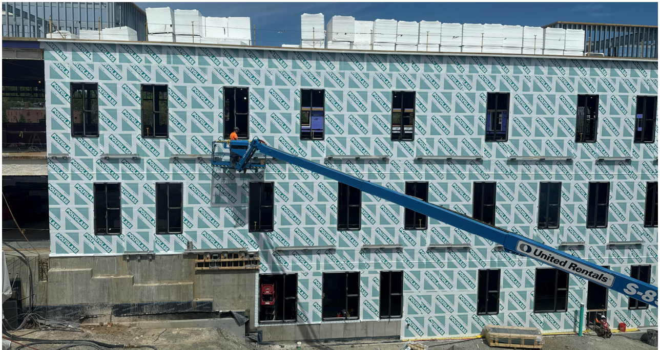
May 26: AVB and Window Installation on East Elevation
