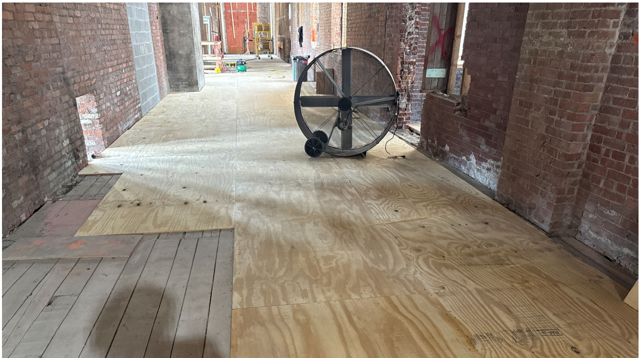
May 14: Plywood in corridor, level 2 Historic Building
