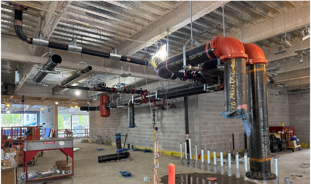
May 26: Mechanical Room Progress
