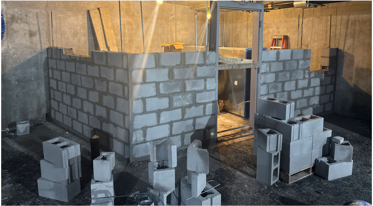
May 20: Water Room CMU Installation
